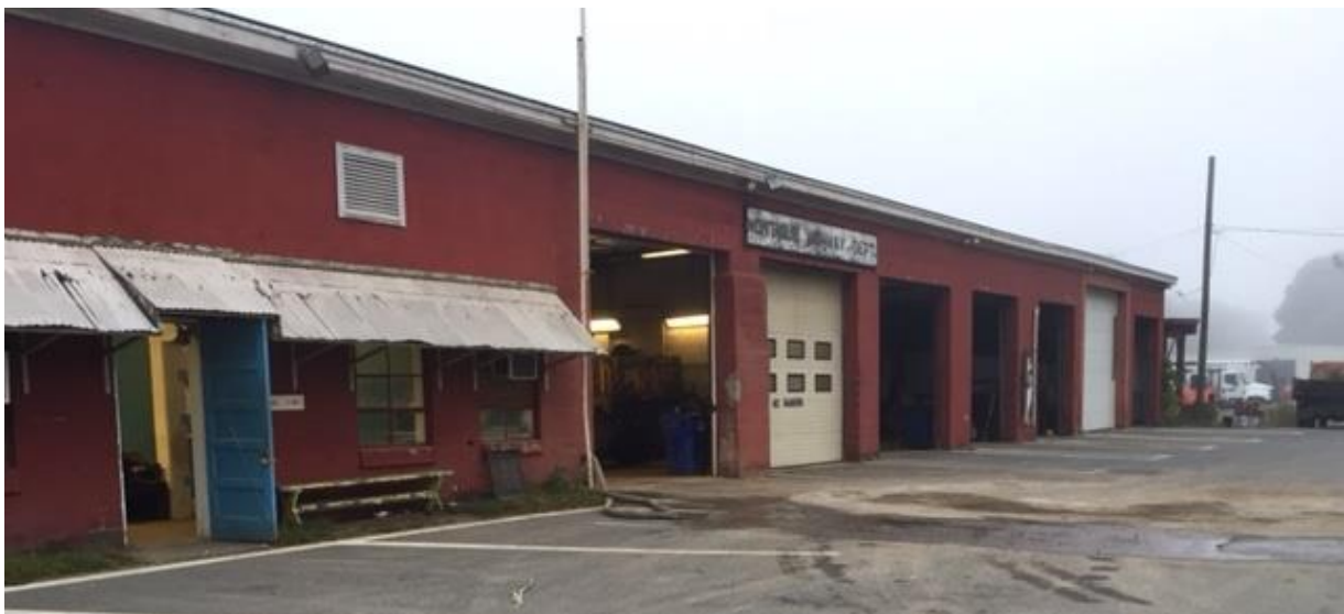
Front of building
