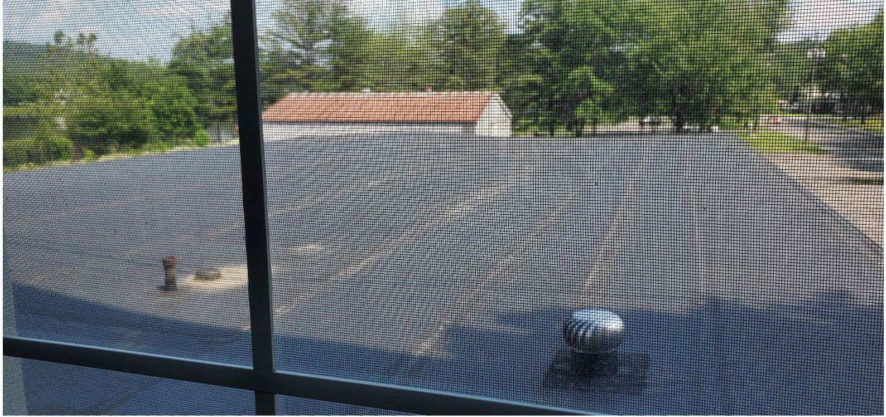
Roof From First Floor of Town Hall looking toward the southeast.
