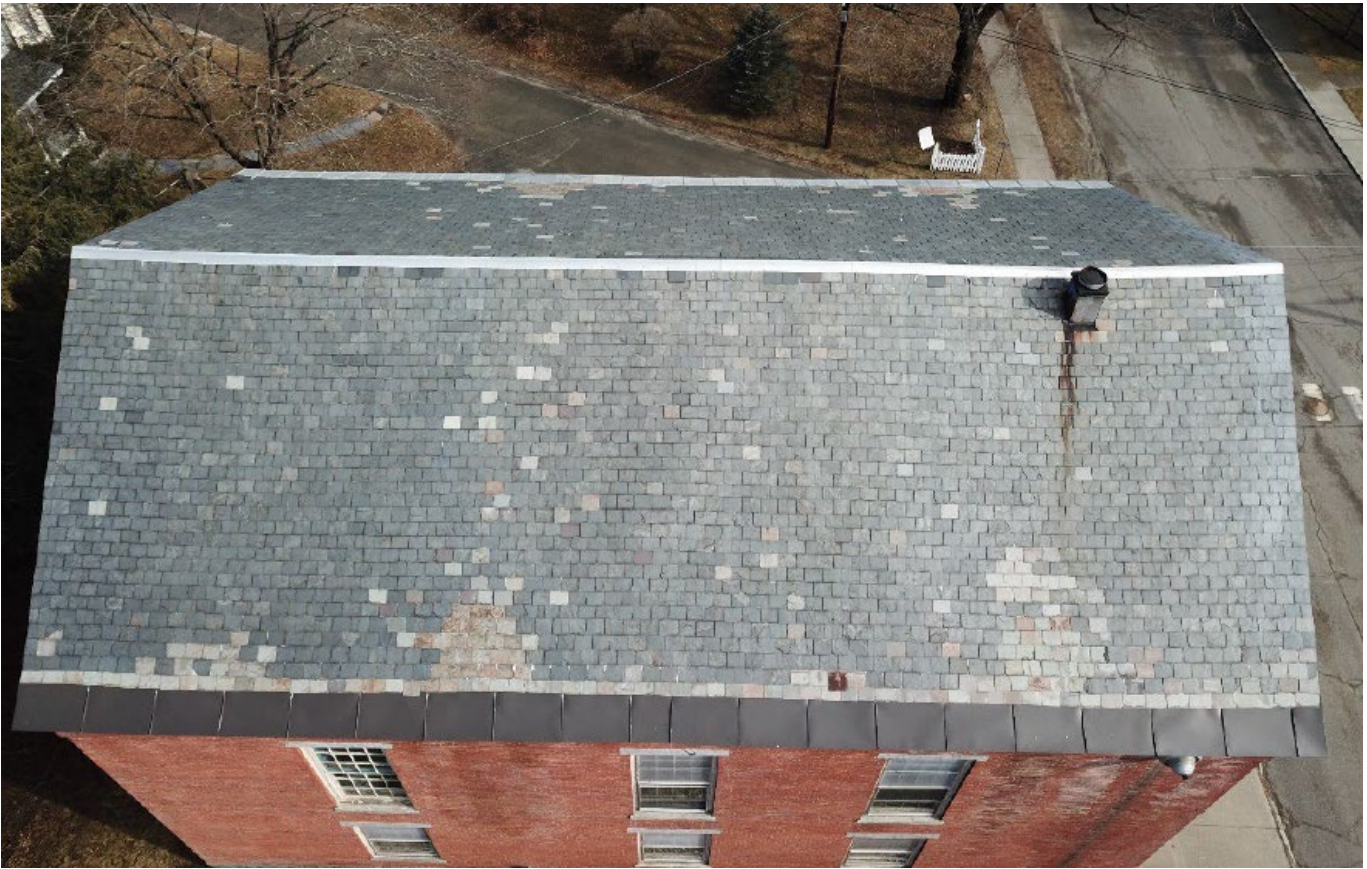
View of the steep sloped slate roof looking west to east.
