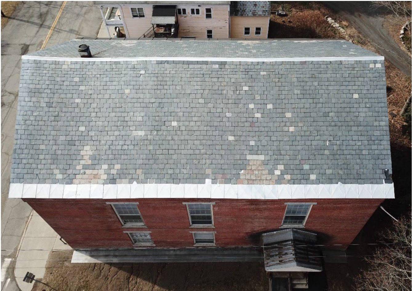
View of the steep sloped slate roof looking east to west.
