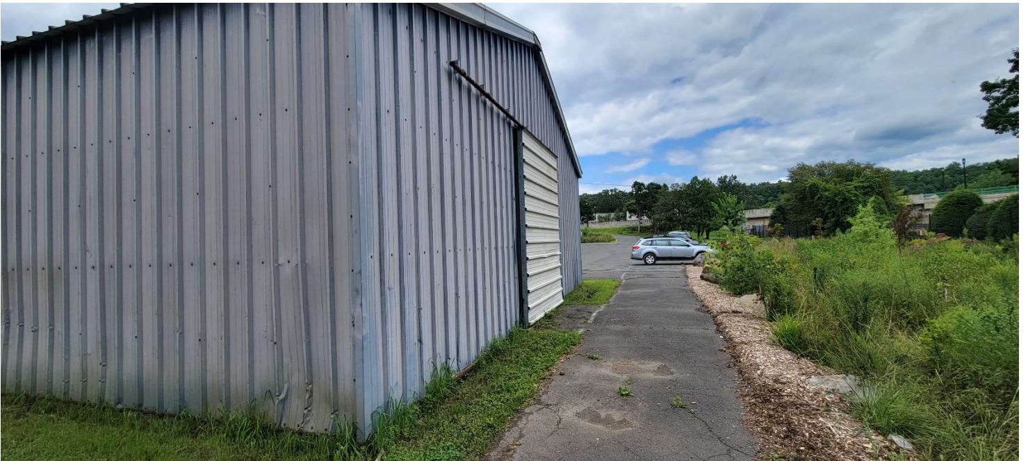
Metal Building Rear Corner Exterior
