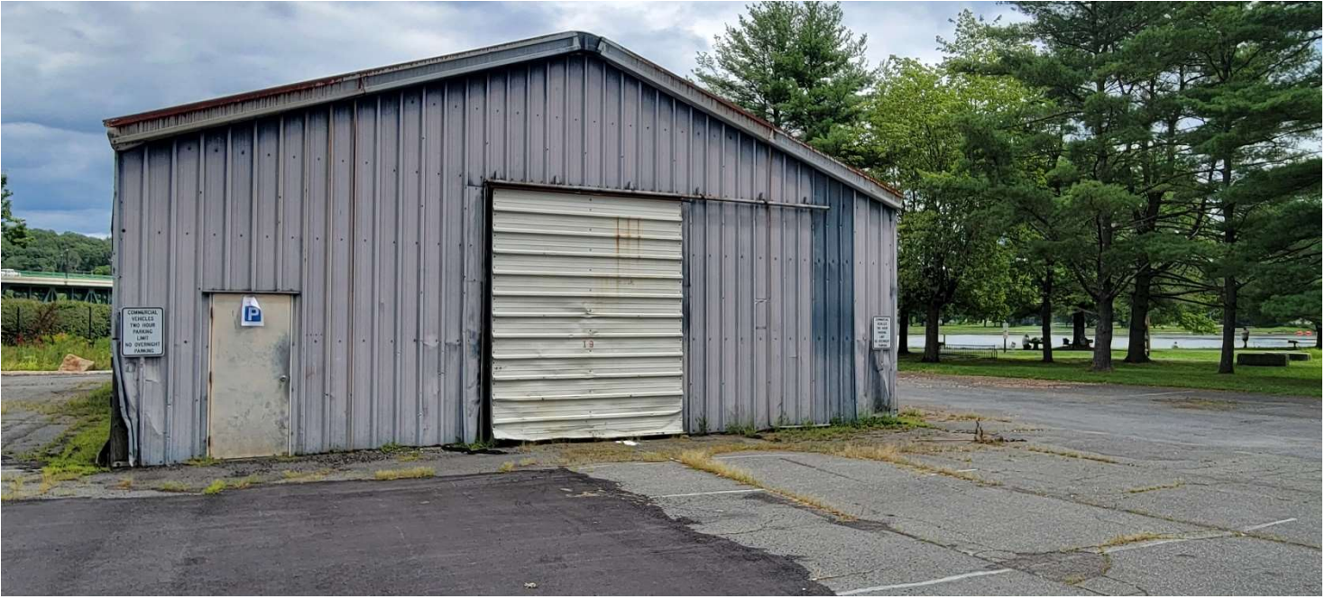
Metal Building Front Exterior
