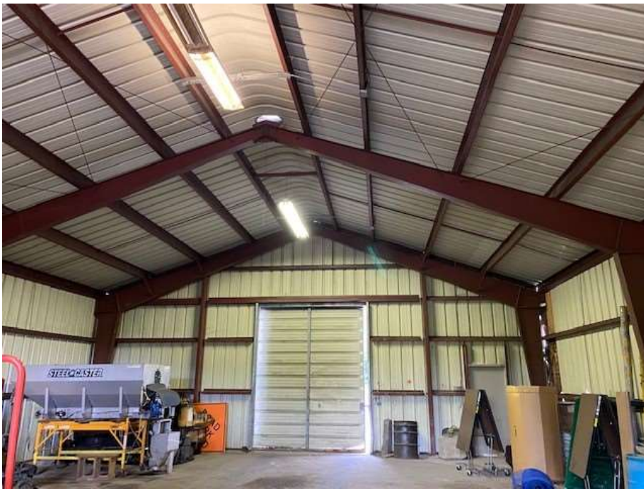
Metal Building Interior (7 photos)
