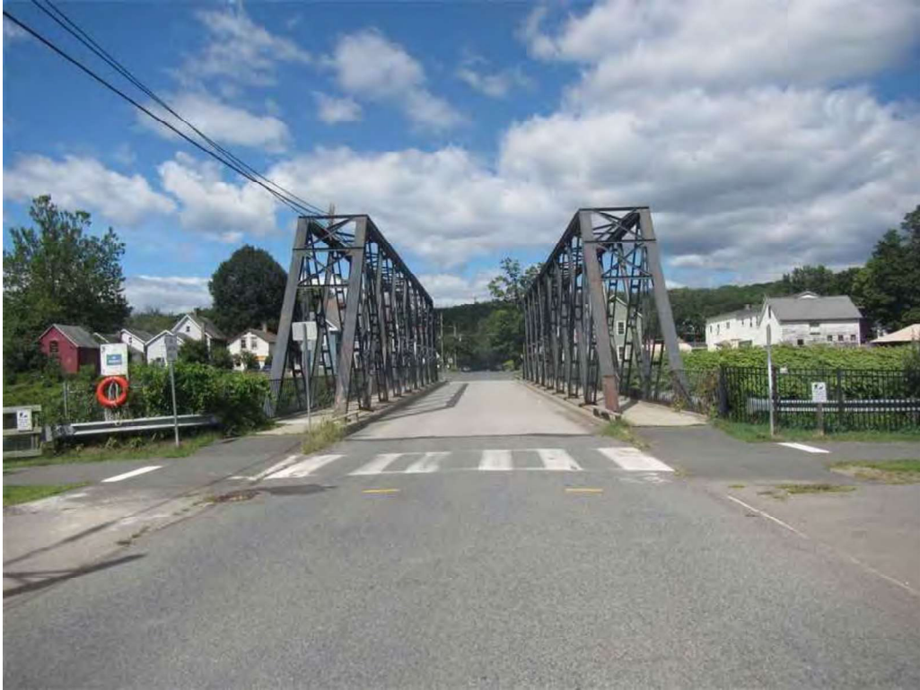
Photo 4: Bridge from east approach.
