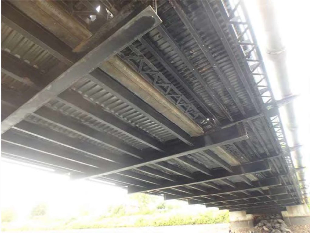
Photo 5: Underside of deck and superstructure, span 2 shown, looking west.
