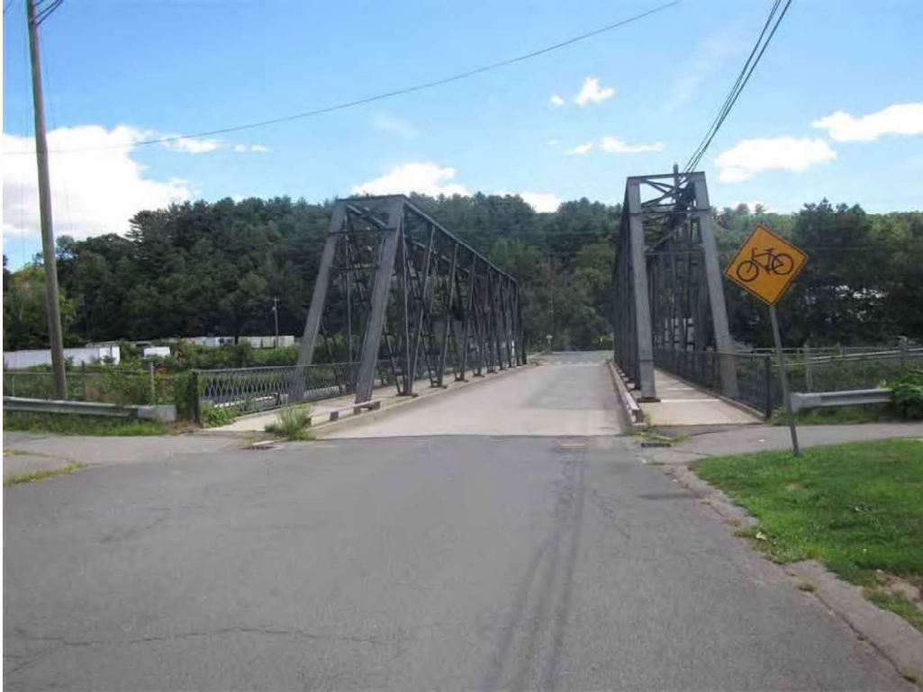
Photo 3: Bridge from west approach.
