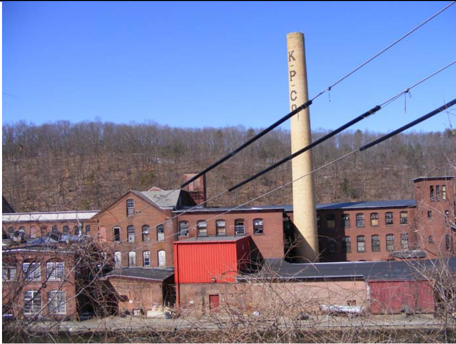
2014 View of South Elevations (Source: TRC)
