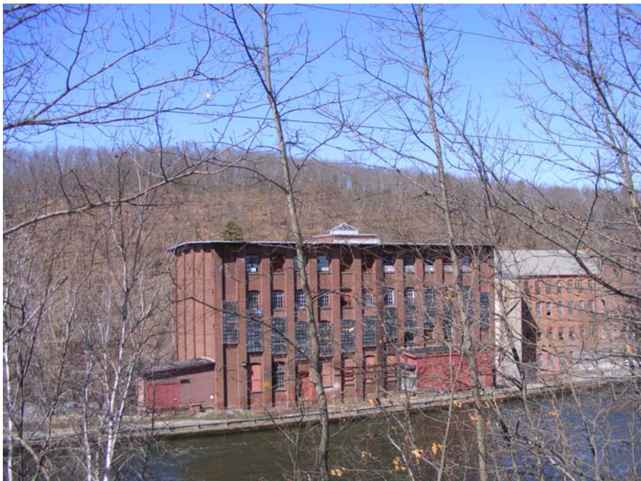
2014 View of Southern Storage Building (Source: TRC)
