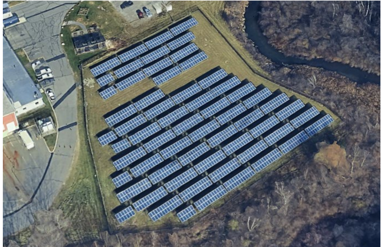
Image of 1 MW ground-mounted solar system in Pittsfield, MA. Photo credit: Google Earth
