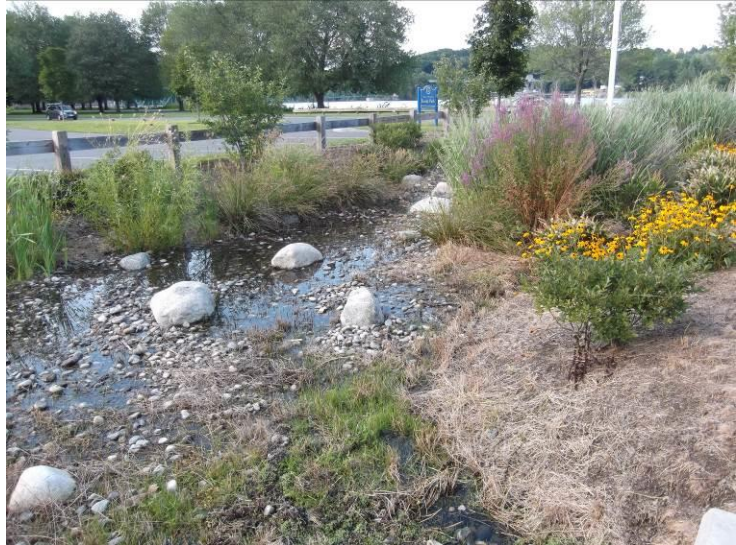
An example of Low Impact Development (LID) stormwater management at Unity Park. A rain garden treats stormwater runoff from the parking area and the playground water feature.
