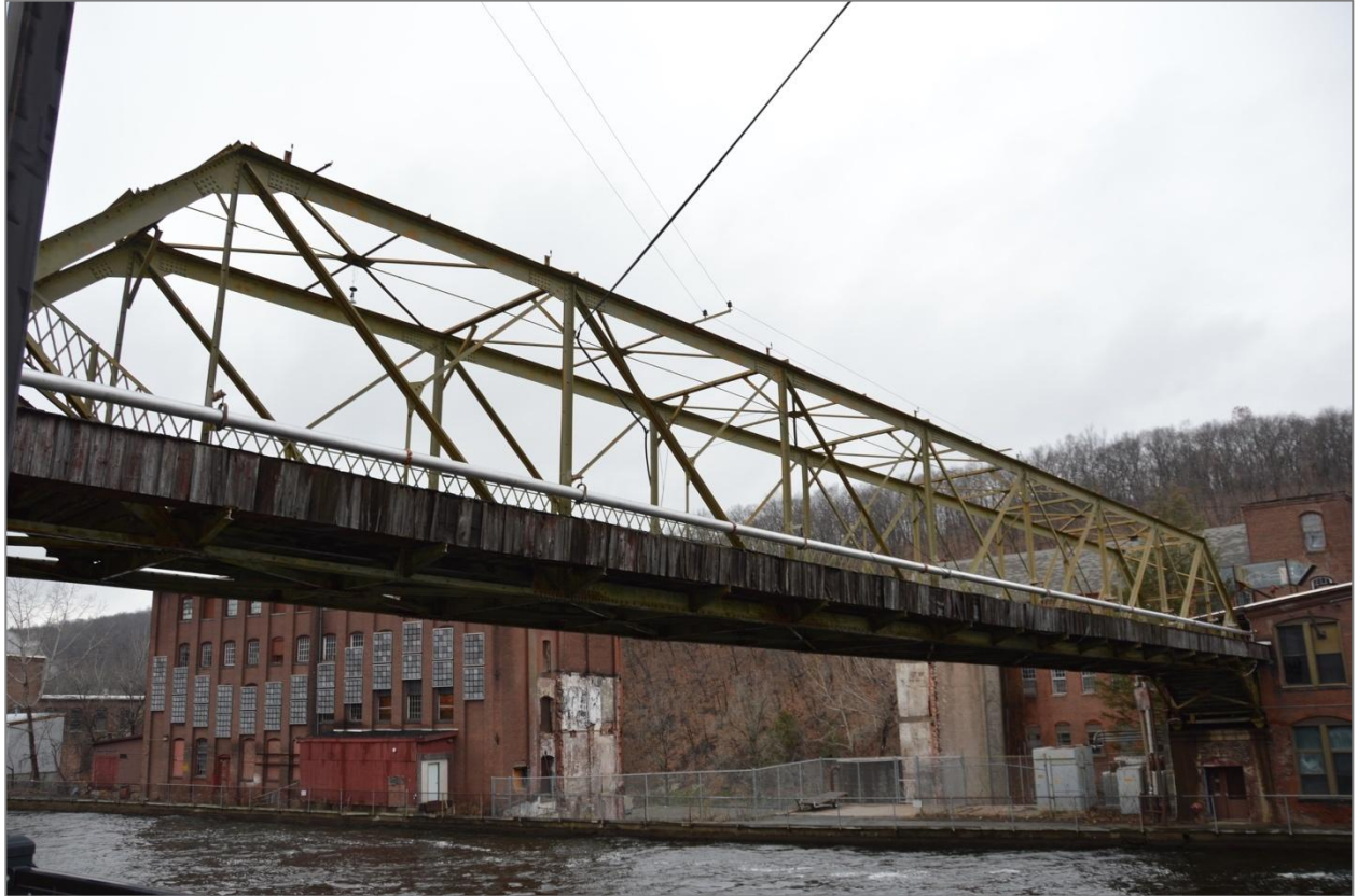
Figure 67. The Strathmore Pedestrian Bridge carries sewer and water infrastructure to the District
