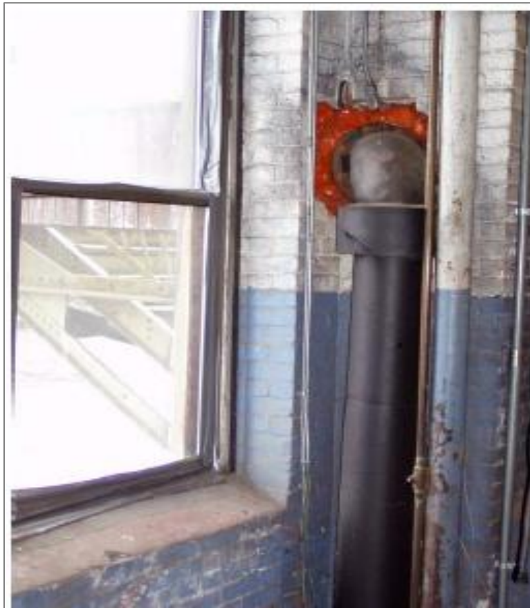
Figure 103. 6- 8" inactive water main from Strathmore Pedestrian Bridge entering Building 4 (Fuss & O'Neill)
