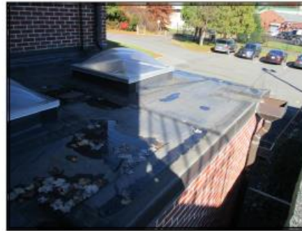
Photo R27 — View of EPDM roofing system on rear entrance roof.
