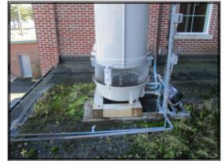
Photo R30 – View of equipment room roof at cooling tower with heavy moss and vegetative growth.
