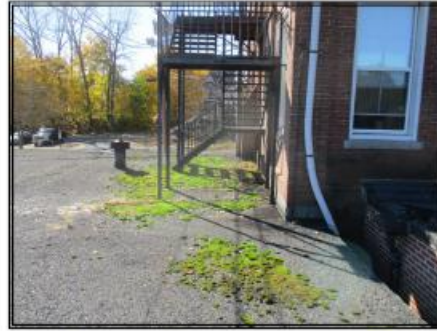
Photo R19 — View of stair tower and moss growth on built-up roof at garage roof..
