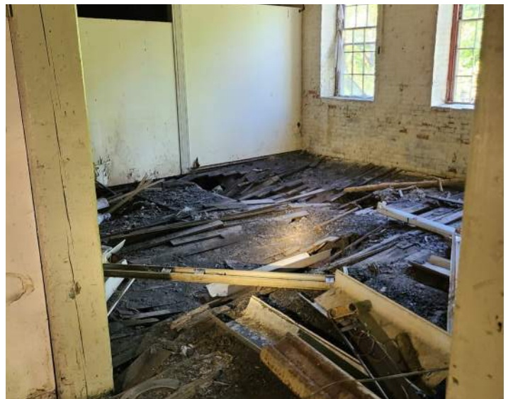
6 Building 1 Collapsed Floor System
