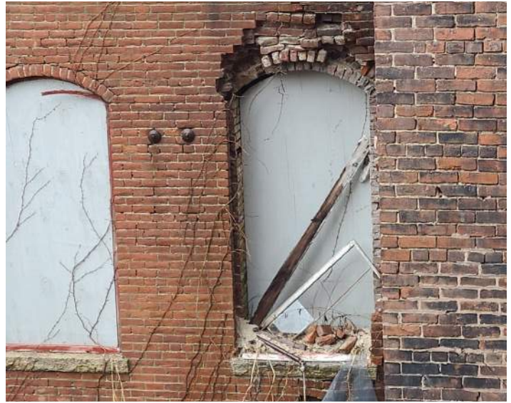
2 Building 1 Failing Window Arches
