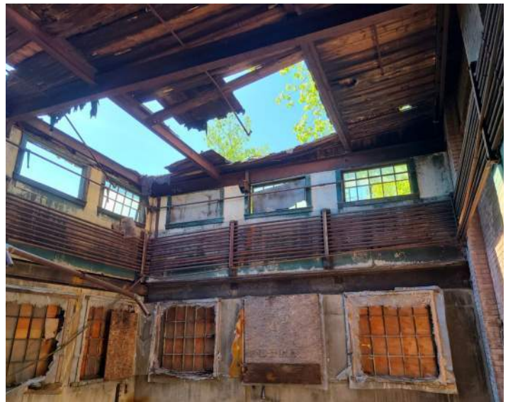
4 Building 11 Addition Collapsed Roof
