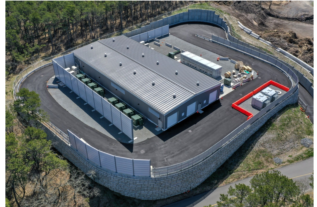
Image of a 38 MWh commercial battery storage system based in Provincetown, MA. The facility stands on a paved lot and is surrounded by forested land. Photo credit: Eversource
