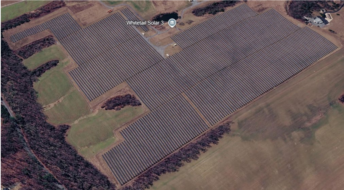
Image of an expansive 20 MW commercial ground-mounted solar in Franklin County, PA. Photo credit: Google Earth
