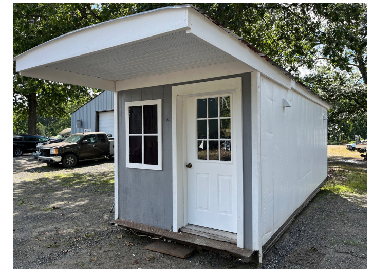
Image of Temporary Shed see plan Shed shall be: 24 ft. L x 8 ft. W as shown in the photos
