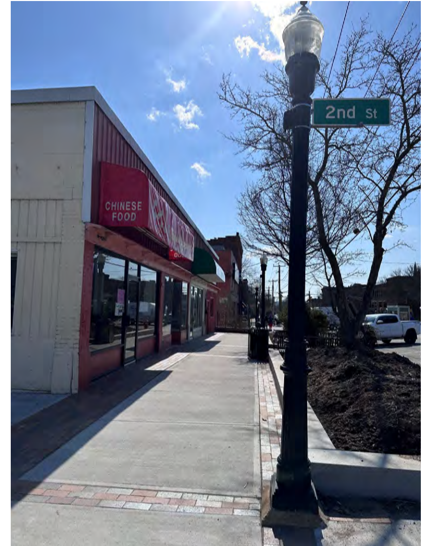
Figure 3: Photo shows completed Ave A block in front of CeCe's Chinese Restaurant, Subway, and Breakdown Records
