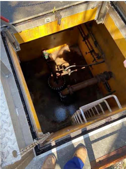
Current Dry Pit Diaphragm Pump, Check Valves
