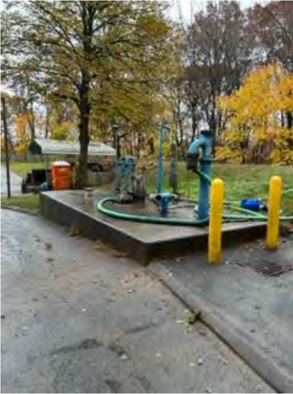
Current Receiving Station Manual Screen Only
