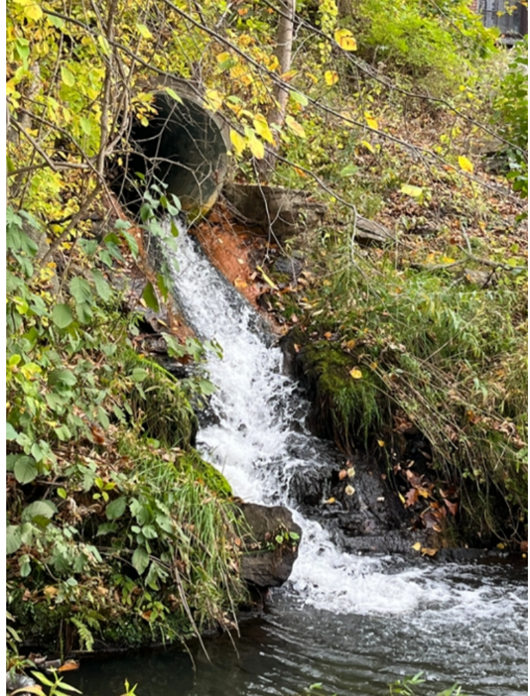
Outfall 02: Adjacent to Power Canal
