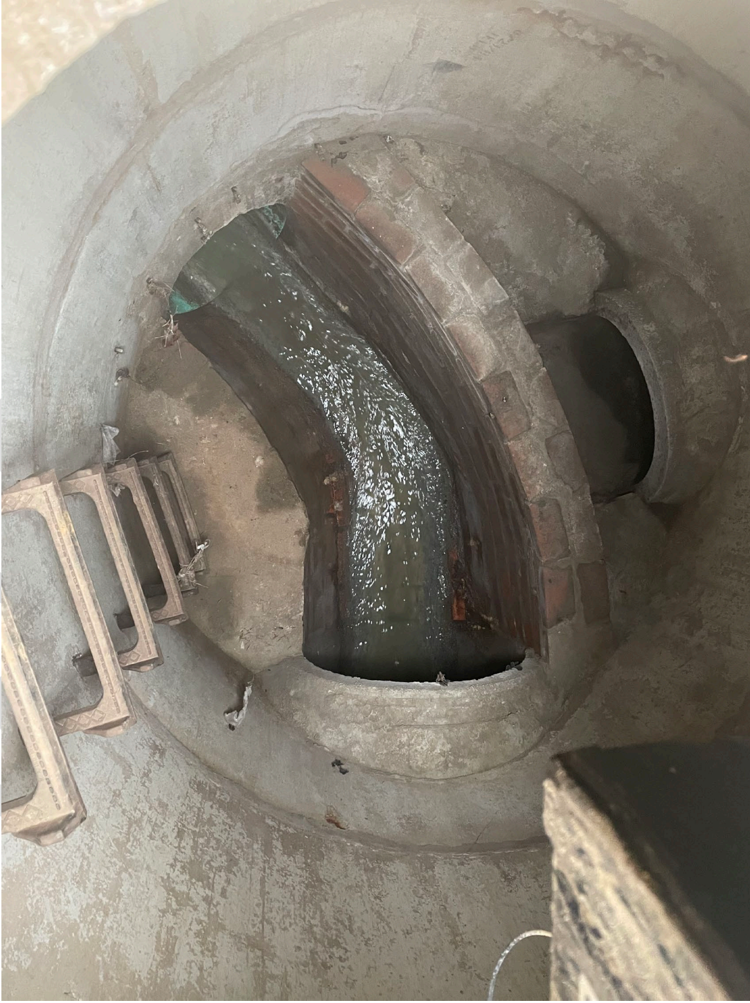
Photo 1: Avenue A Overflow Weir Manhole #AV-13
