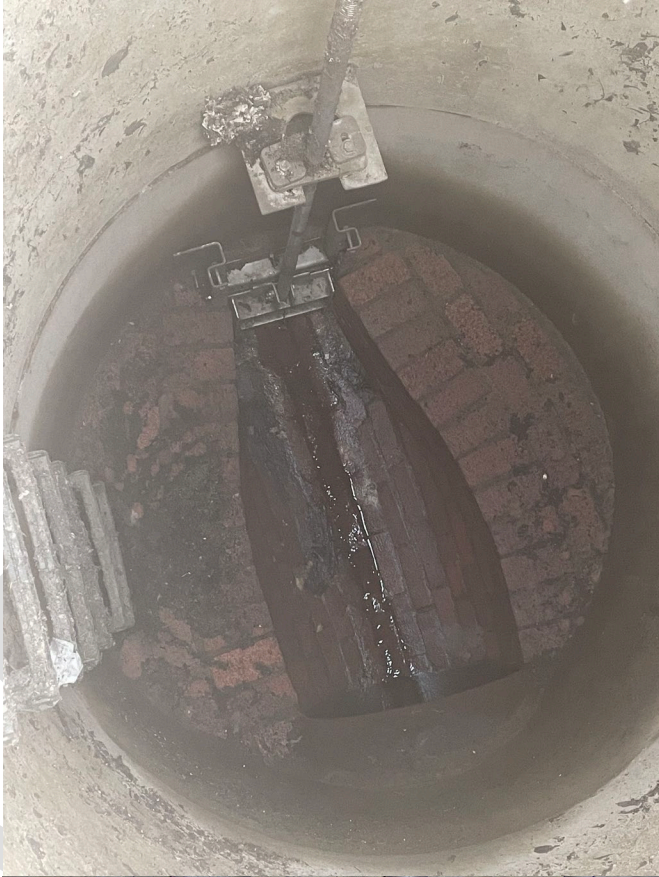
Photo #2: Avenue A Gate Manhole # AVP-3
