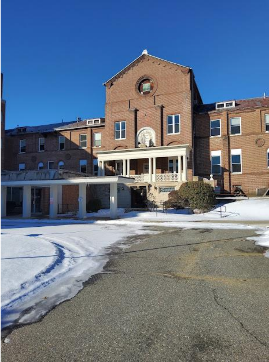
3 of 3 East Elevation of Main Entrance
