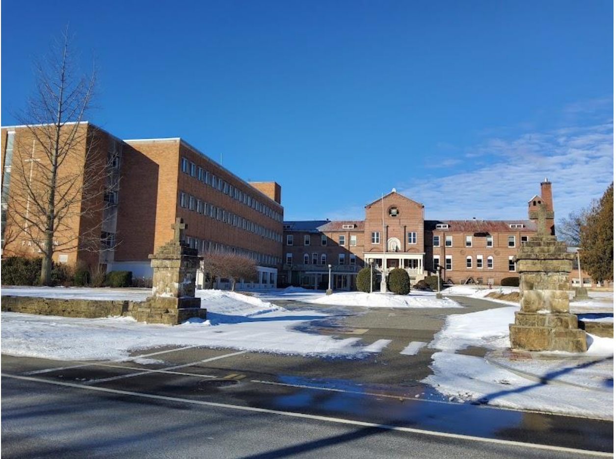
1 of 3 East-facing elevation of Original Building with non-contributing addition
