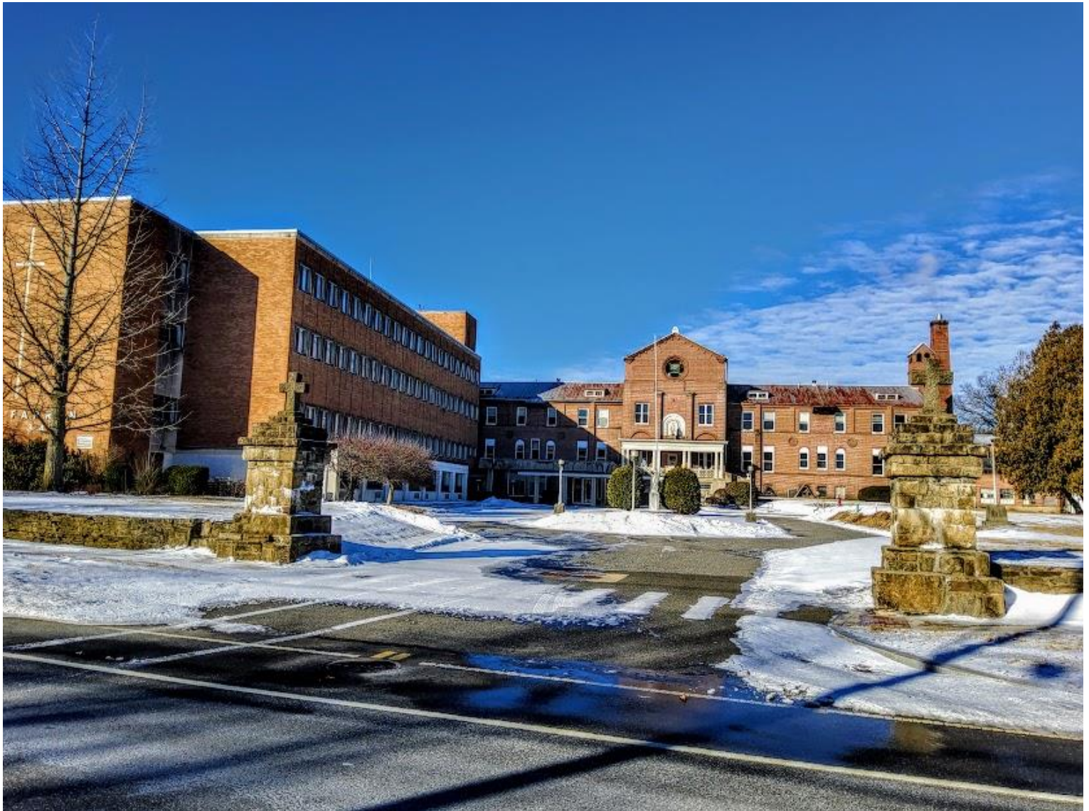
February 2022 photo of entire complex. East elevations.
