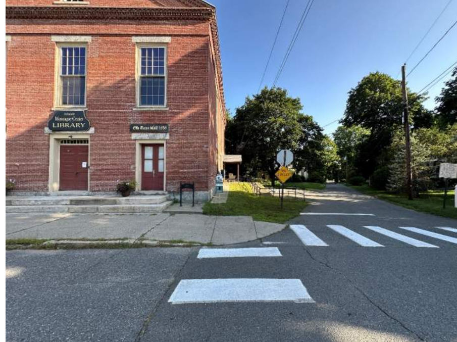
OUTDATED PEDESTRIAN CURB RAMPS
