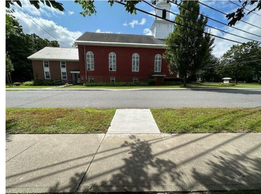
NO CROSSWALK MARKINGS OR SIGNAGE
