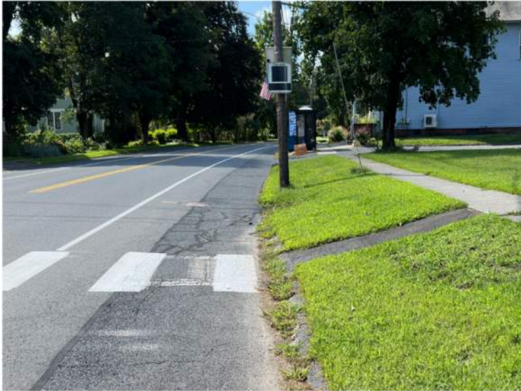
SPEEDING AND STEEP CURB RAMP TO SIDEWALK
