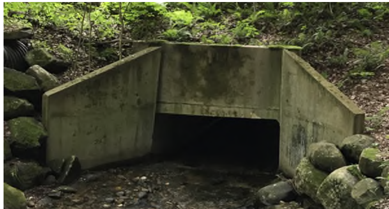
Culvert 2149i on Ripley Road:
