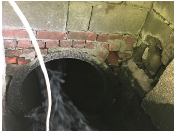
Culvert 1871i at School Street and Station Street:
