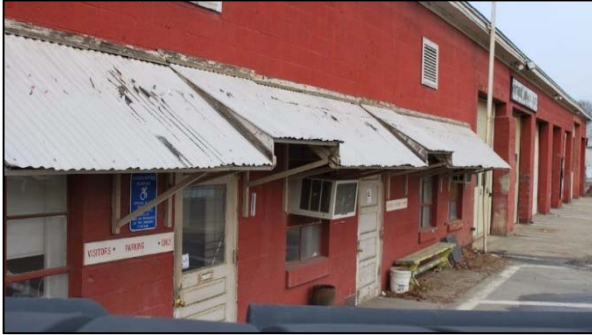
Figure 70. View of DPW facility
