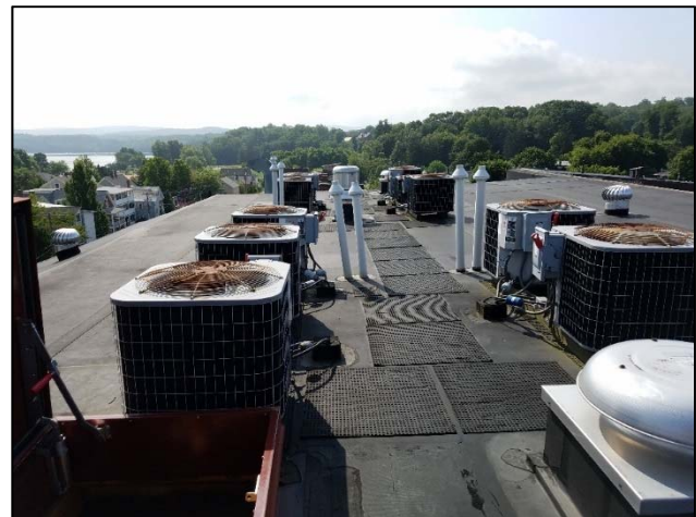
Figure 63. Ten separate units on Colle Building rooftop
