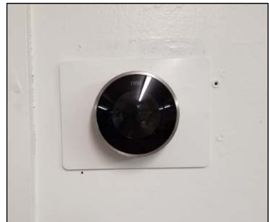
Figure 48. Remotely adjustable thermostat
