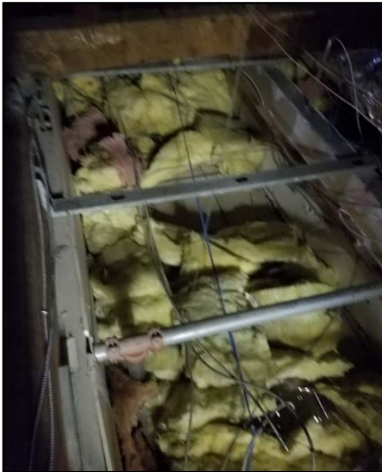
Figure 66. Roof insulation configuration
