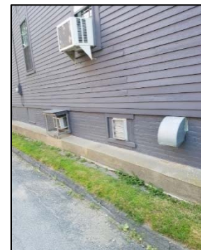
Figure 45. AC units on western side of building
