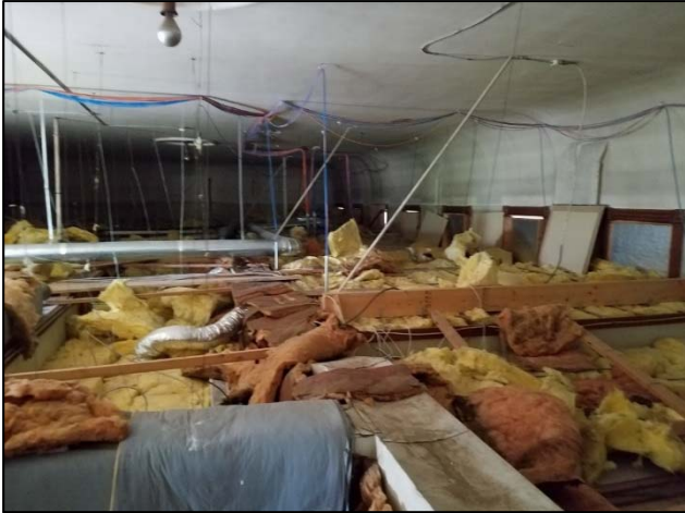
Figure 52. Condition of attic insulation
