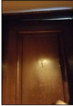
Figure 18. Doorway to employee offices in basement with large air gap
