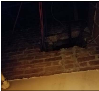
Figure 55. Additional wall gaps in basement
