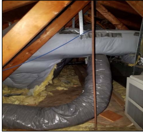
Figure 11. Uninsulated Ductwork
