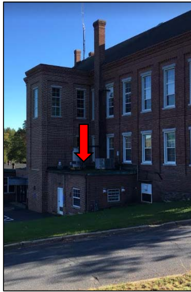
Figure 50. View of boiler room
