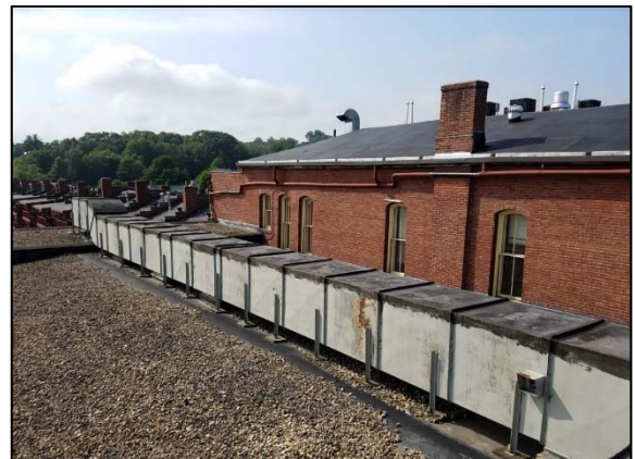
Figure 62. Original HVAC ductwork scheduled for replacement
