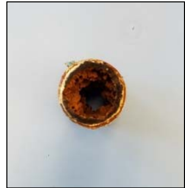
Figure 36. Removed piece of piping from Hillcrest illustrating impact of hard water.
