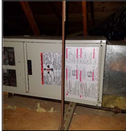
Figure 13. Airport building furnace
