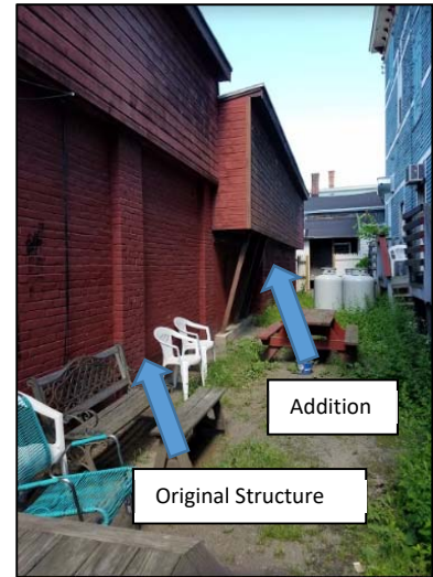
Figure 22. View of Library from adjacent apartment seating area
