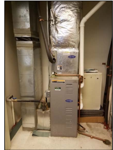
Figure 67. One of 10 Individual furnaces
