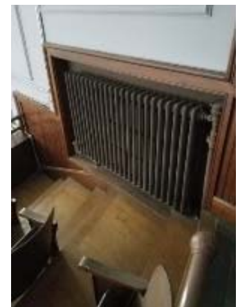
Figure 38. Auditorium radiator in balcony
