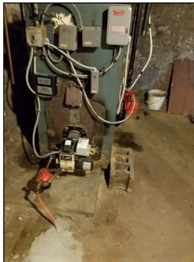
Figure 27. Inadequate boiler with unused components
