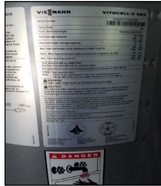
Figure 56. VIESSMANN indirect fired domestic hot water storage tank
