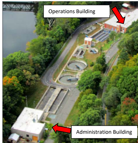
Figure 68. Aerial view of WPCF
