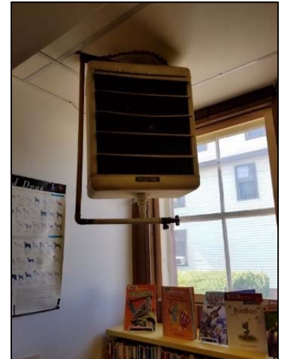
Figure 26. Hydronic unit heater
