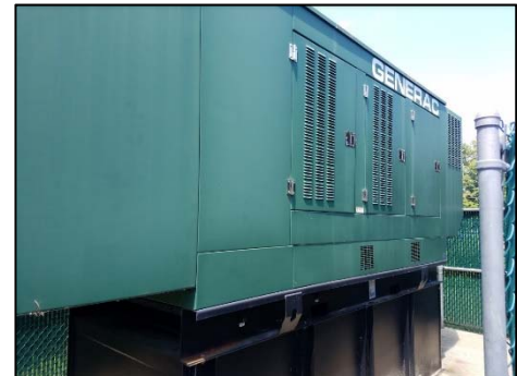
Figure 42. Public Safety Complex diesel generator
