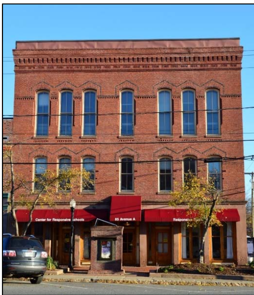
Figure 64. View of Colle Building from Avenue A
