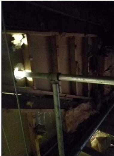
Figure 65. Visible light through insulation
