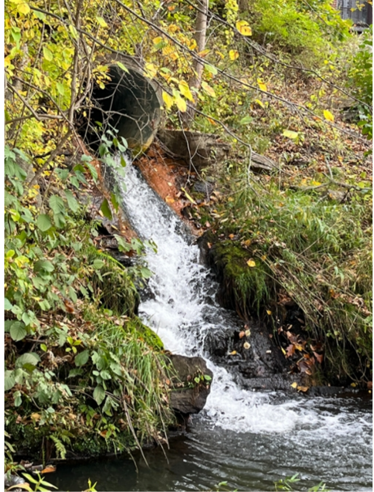
Outfall 02: Adjacent to Power Canal
