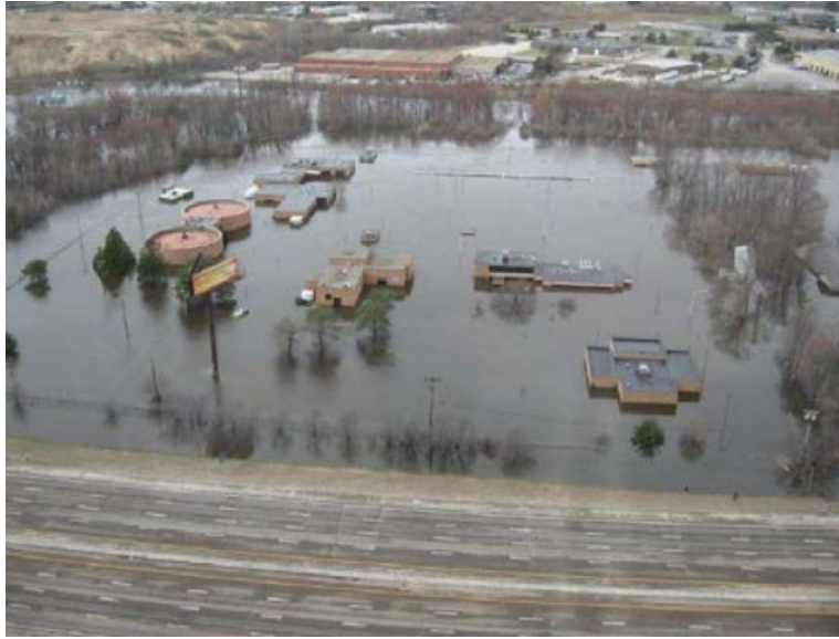
Figure 1: The flooded Warwick wastewater facility on Wednesday, March 31, 2010. (State of Rhode Island)
