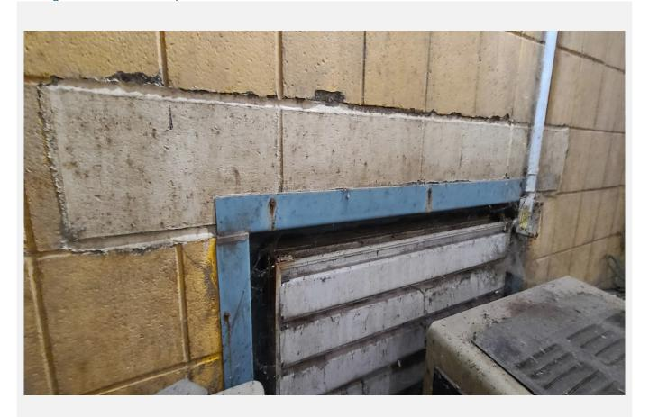
Existing Low Point Exhaust Ductwork, Grille, and Explosion Proof Electric Unit Heater
