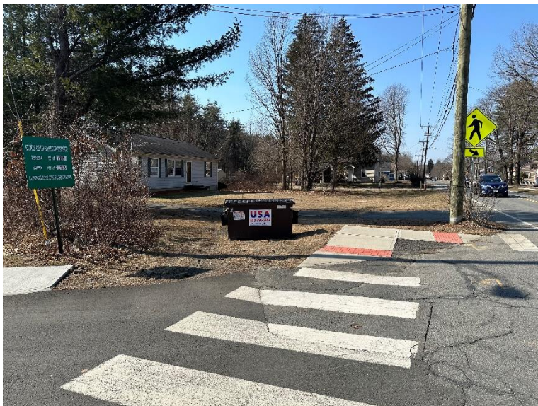
Figure 1: Sandy Lane sidewalk, missing sidewalk section. Photo taken on February 26, 2024
