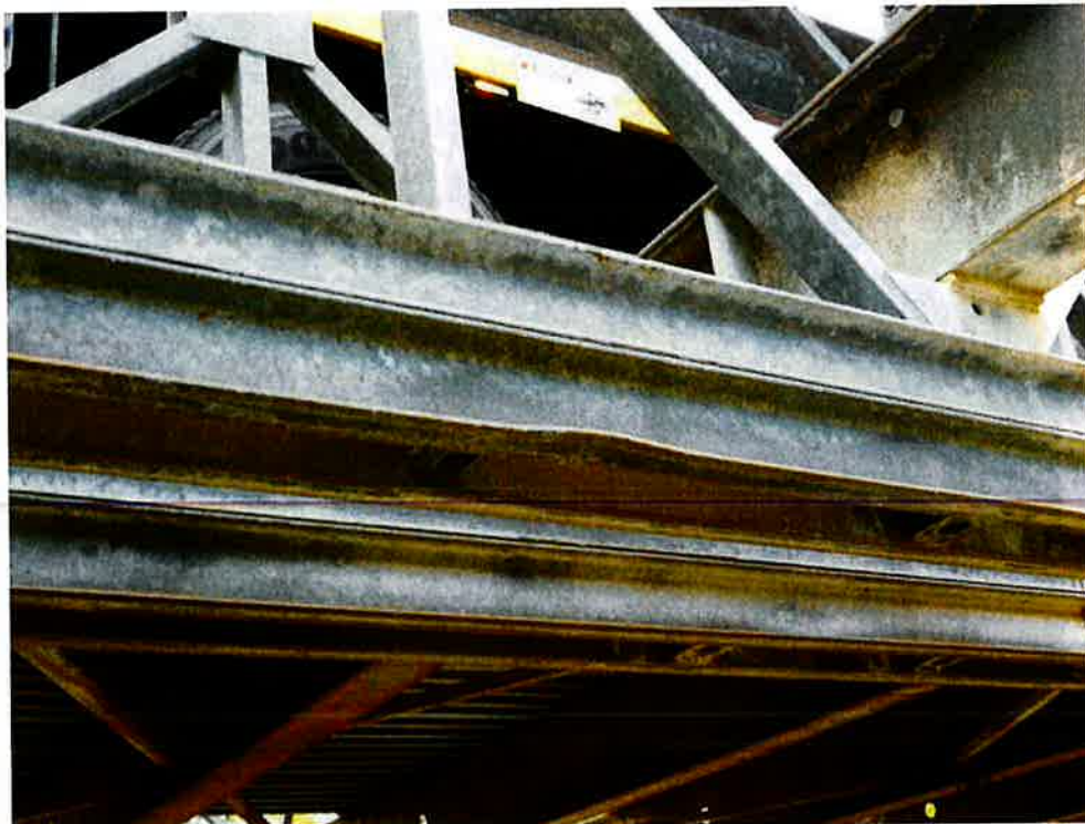
Photo 8: Lower Cord has a few small dents scattered throughout the bridge.
