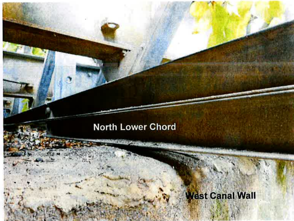
Photo 11: North Truss, Lower Chord, West Abutment, is almost in contact with the top of the canal wall, leaving only 1/2" of clearance.
