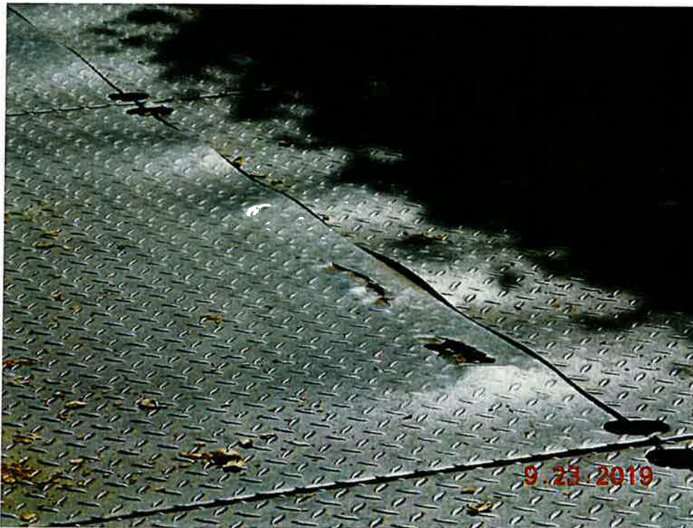
Photo 2: Steel Deck Panels have some pack rusting, between top flange of the fascia joints and steel panels. A few Deck Panels have through holes near the outer edges of the panels.
