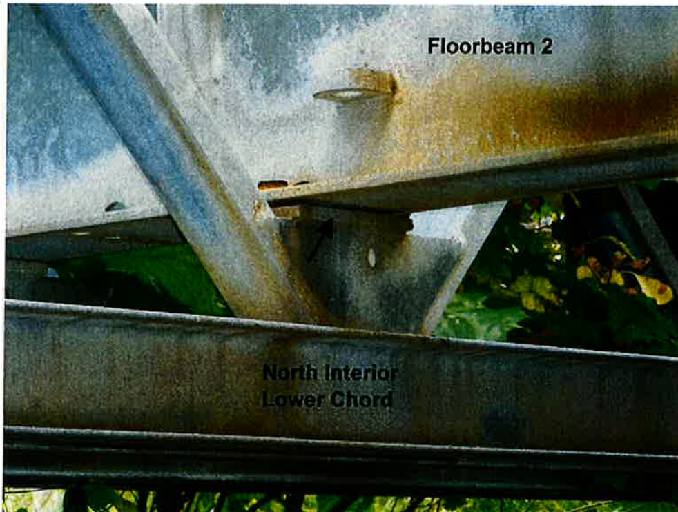
Photo 6: Some Floorbeams, are slightly lifting up from Floorbeam Bracing System. Floorbeam Bracing System has areas of light rust staining.
