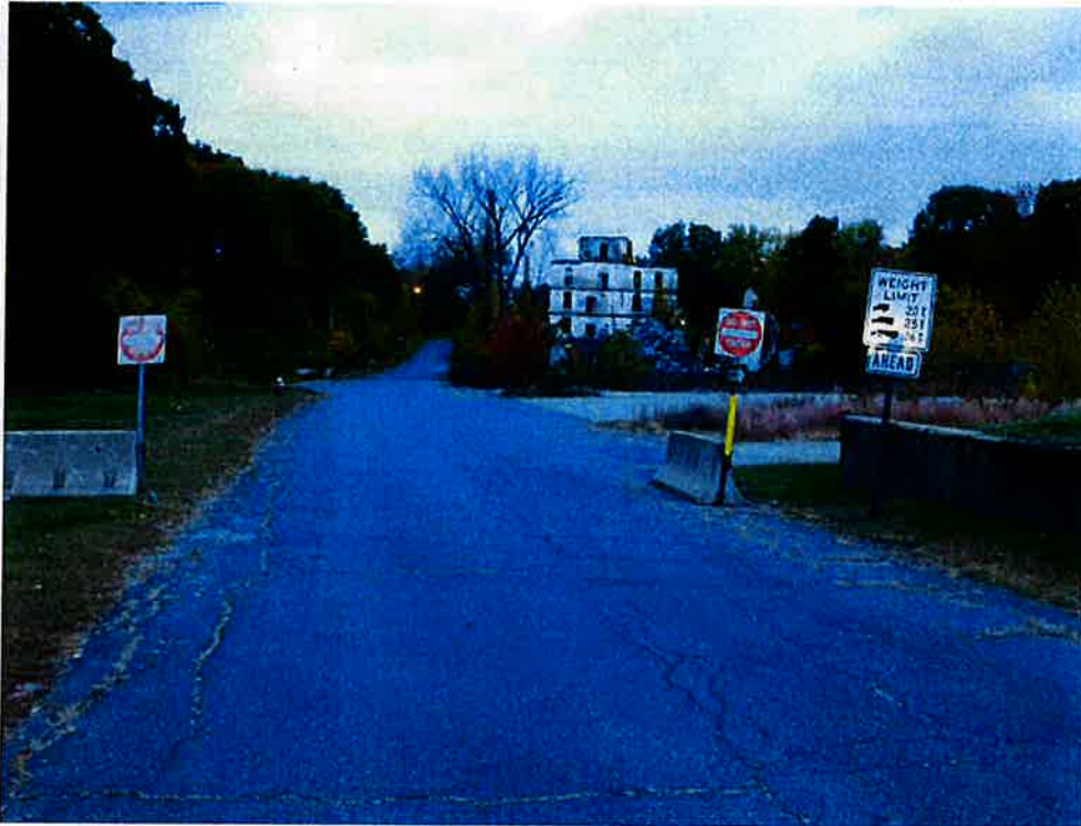
Photo 1: West Approach, has two "DO NOT ENTER" signs along with a "Advance" Weight Posting.
