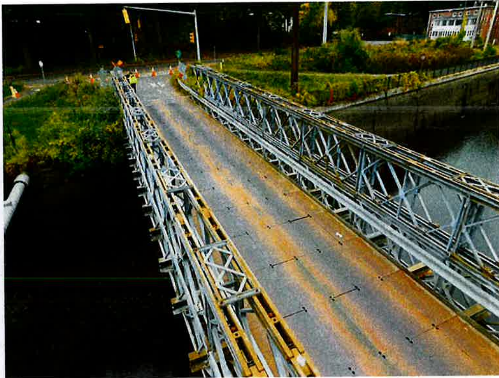
Photo 7: Top surface of Upper Chords have areas of light rust staining.
