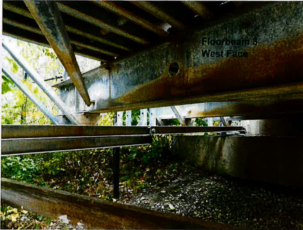
Photo 5: Floorbeams have areas of minor surface rust. West Abutment is undermined.
