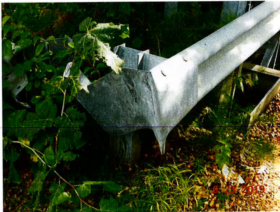
Photo 16: Northwest Approach Guardrail End has collision damage at the bridge abutment.
