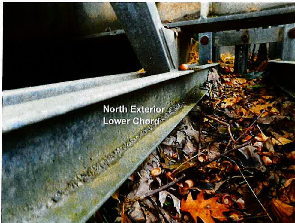
Photo 10: North Truss, Lower Exterior Cord, East Back Wall is "NOT" bent or twisted.
