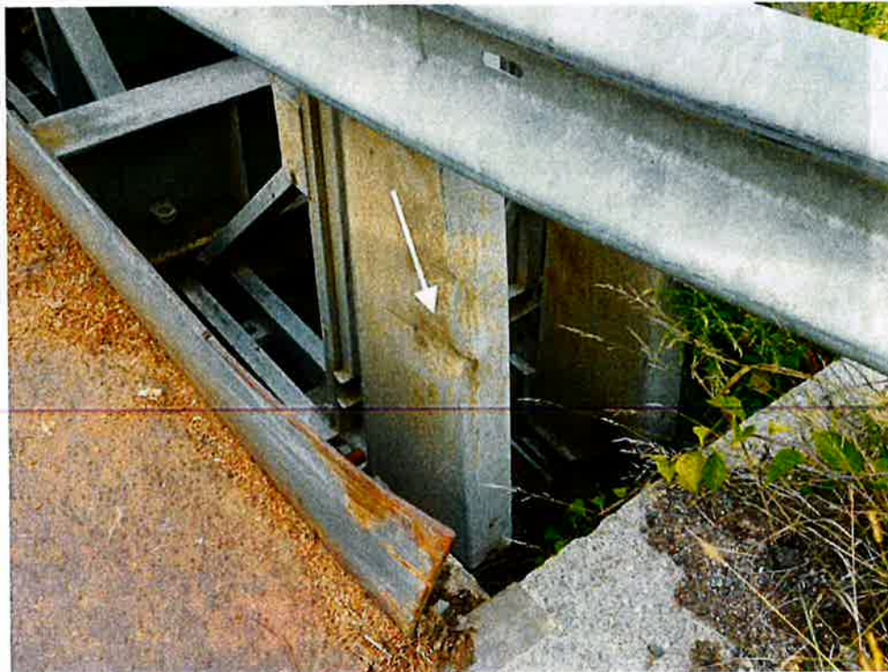
Photo 12: Northeast End Post, interior vertical web member base, is bent from collision damage.
