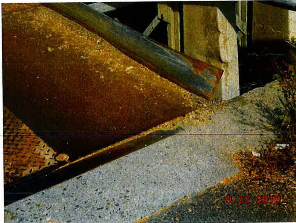
Photo 4: Northeast corner of the Steel Curb is bent due to collision damage.
