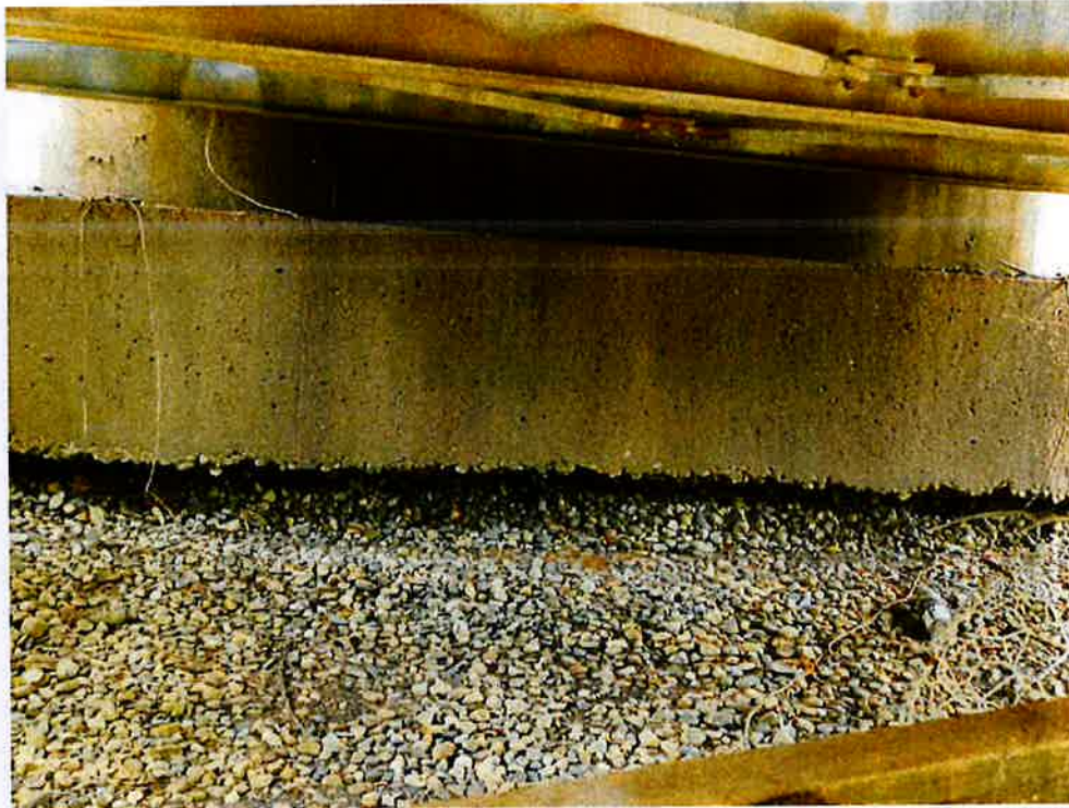
Photo 15: East Breastwall is undermined along the front face with up to 20" penetration.
