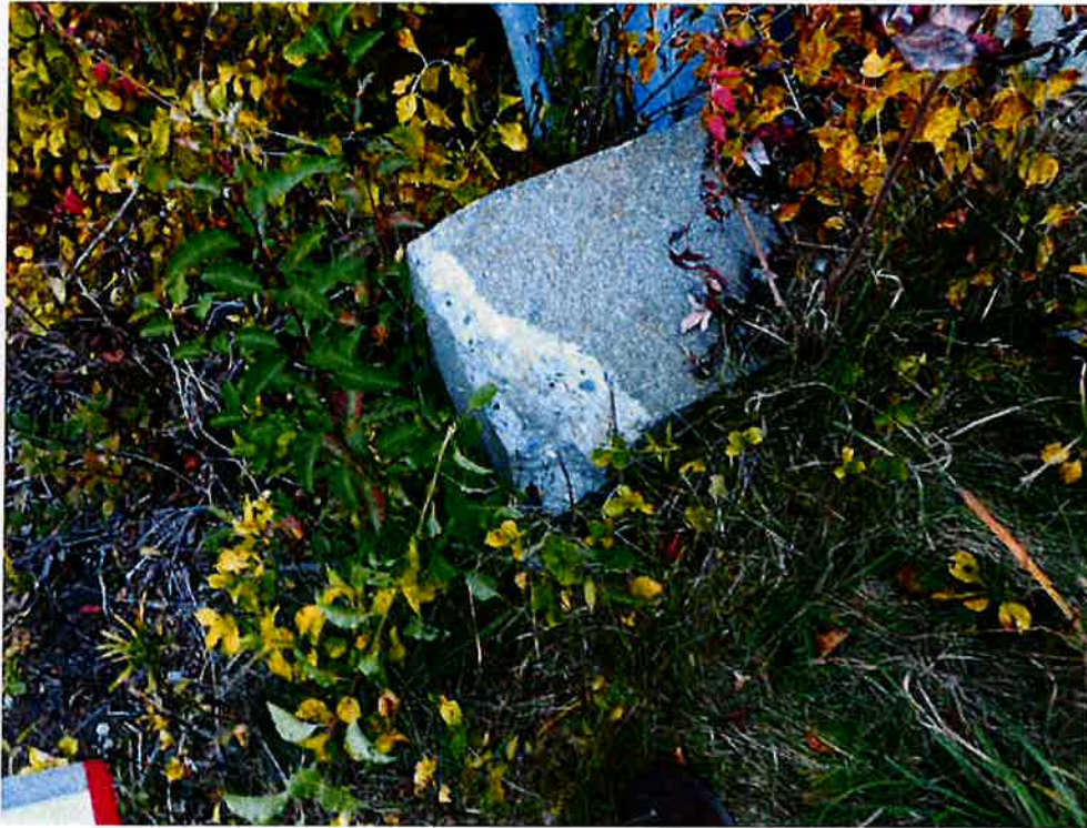
Photo 13: East Concrete Header, South End, is spalled.
