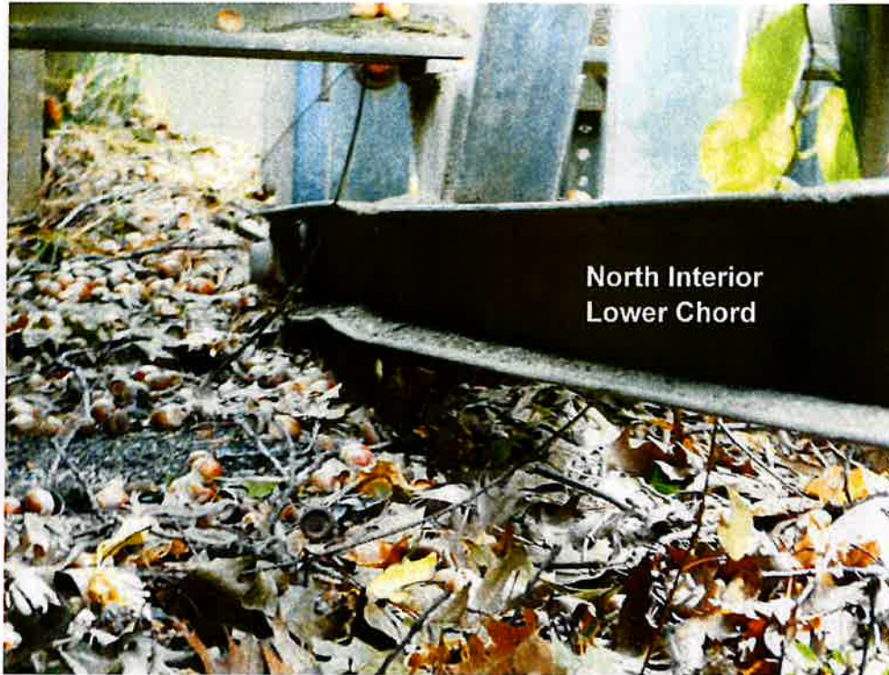
Photo 9: North Truss, Lower Interior Cord, East Back Wall, is bent and twisted. This appears to be from original construction.
