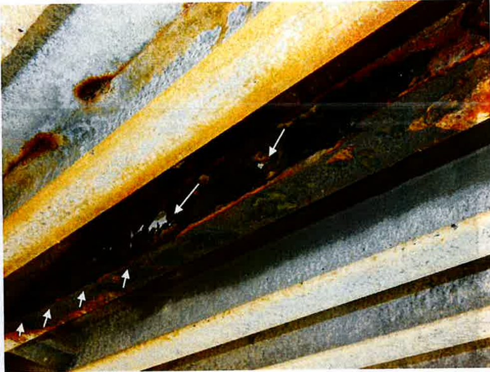
Photo 3: Deck Underside has rust delamination with section loss of some fascia stringers. Stringers have rust holes through the webs and bottom flanges.
