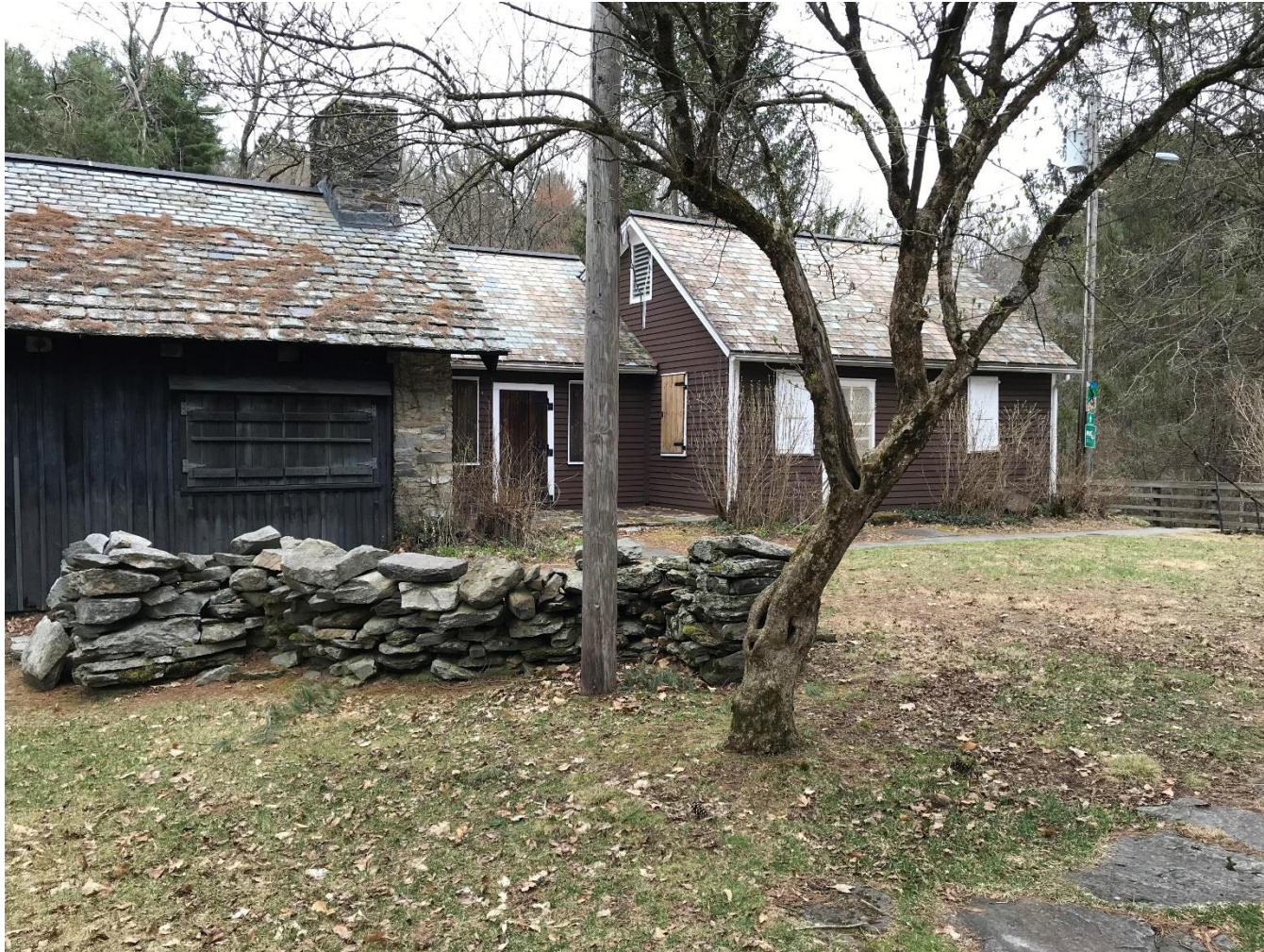
Closed Cabot Camp Buildings April 2019
