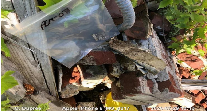
Scene: Suspected ACM Pipe Wrap
