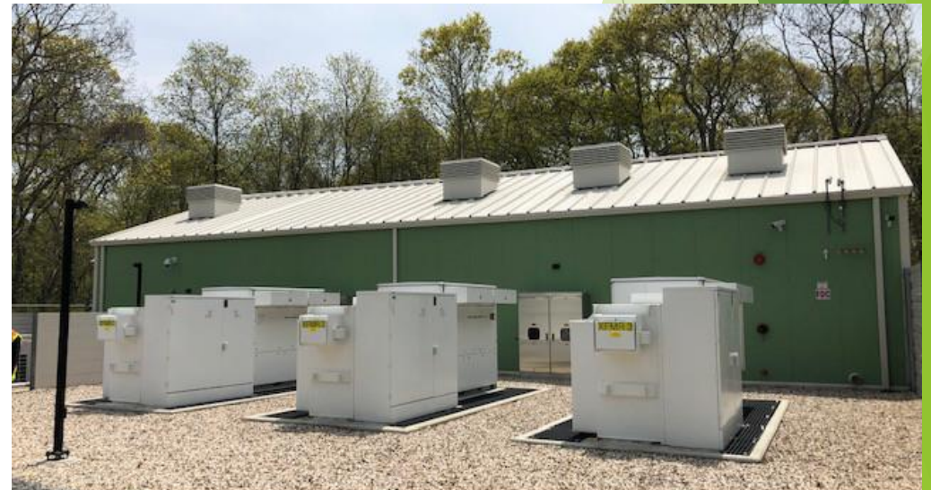
Battery storage facility, East Hampton, Long Island, NY
