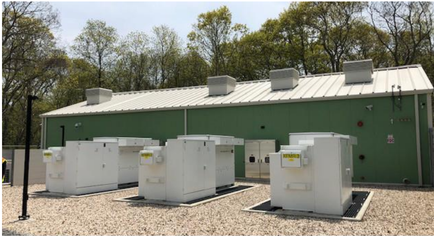
Battery storage facility, East Hampton, Long Island, NY
