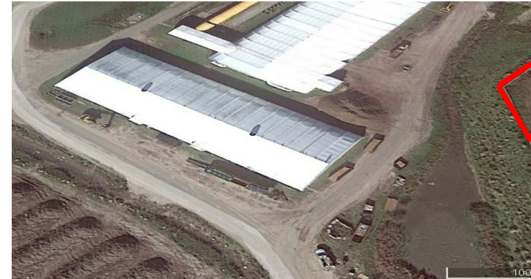
Nantucket Co-Composting Facility 80,000 CFM Biofilter
