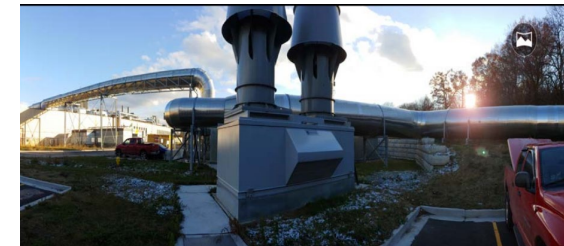
Humber WWTP 30,000 CFM Biofilter Under Parking Lot
