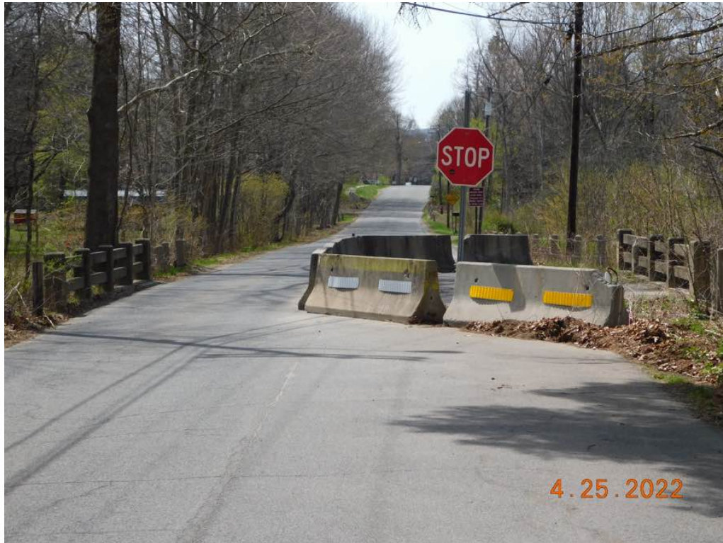
Photo 3: Roadway was restricted with concrete barriers, to 11' wide, off the south curb, taking Beams 1 - 5 out of service. Reflectorized panels are attached to the exterior faces of the concrete barriers.
