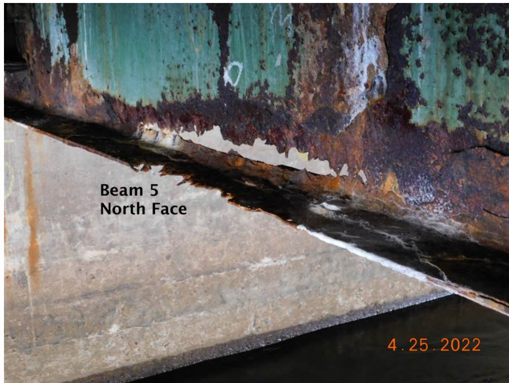
Photo 5: Beam 5 has rust holes in lower web & bottom flange.
