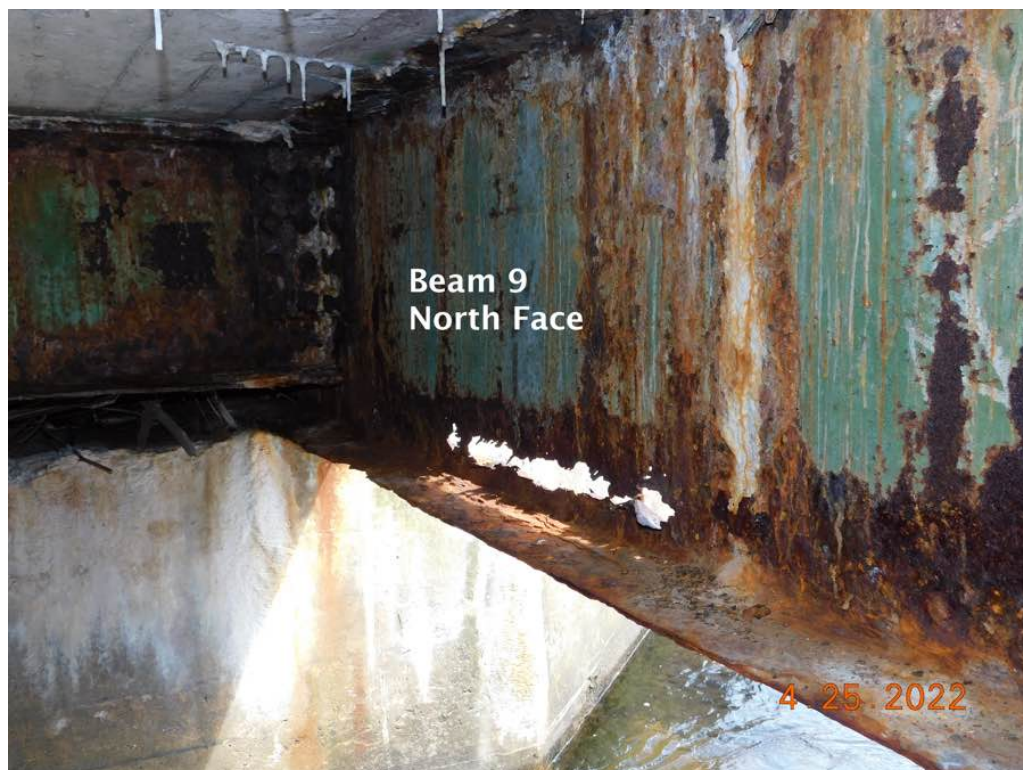
Photo 6: Beam 9 has rust holes in lower web & bottom flange.
