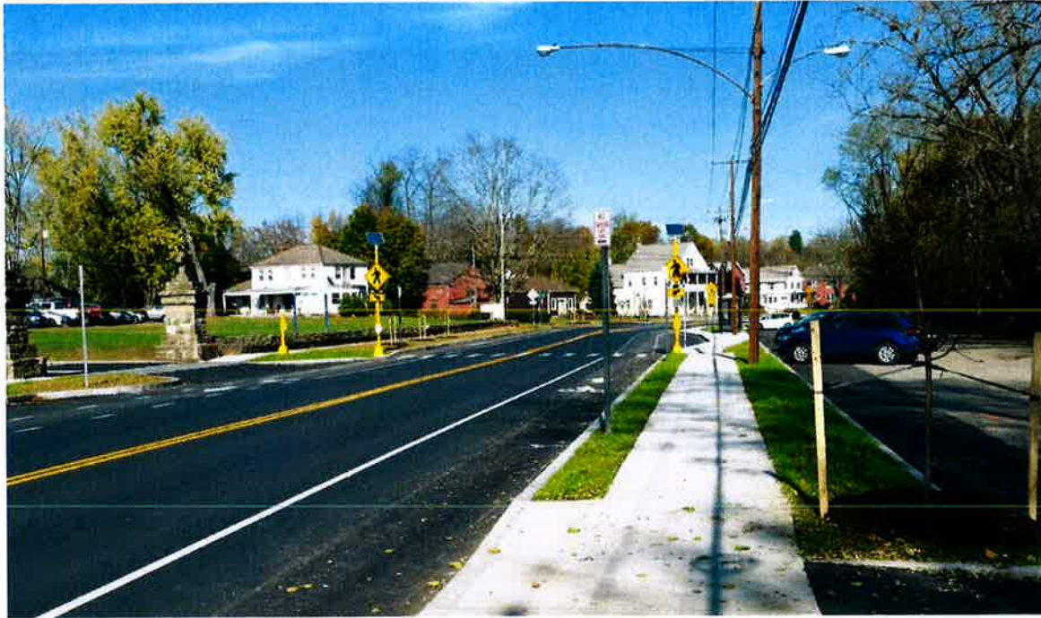
Montague City Road funded by MassDOT TIP in 2016 (project designed by the Town)
