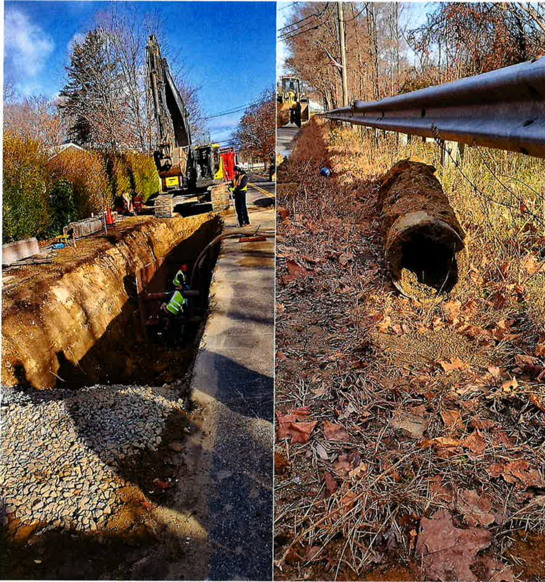
(l) 12 foot deep trenching. Note two drainage pipes are being deployed
