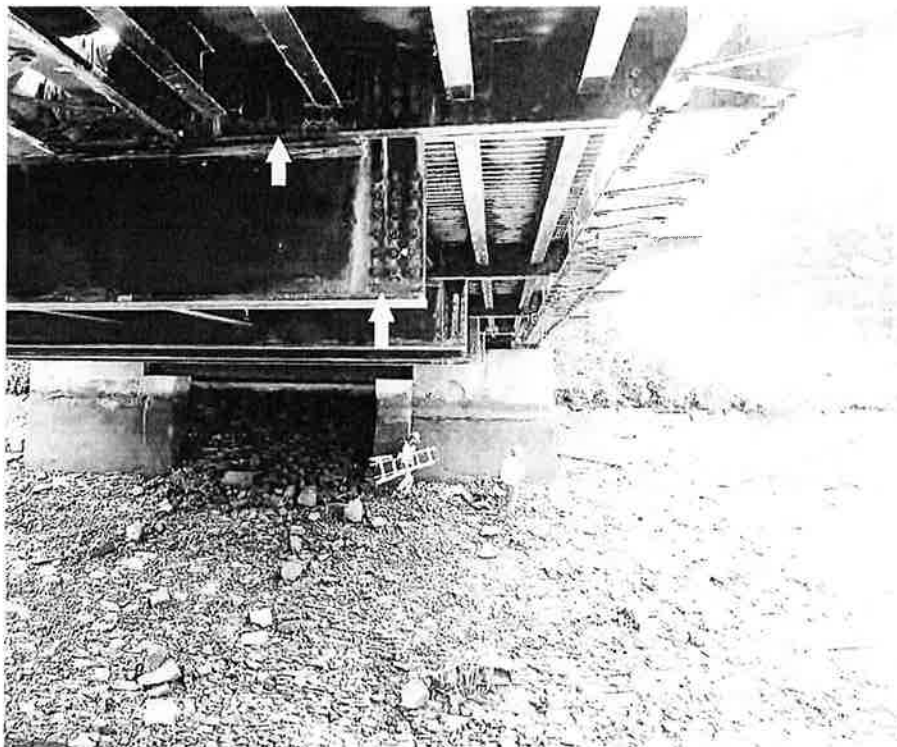
Photo 2: Span 2, floorbeam 6, west face at the south end - sidewalk floorbeam has moderate rust; roadway floorbeam has light rust. Note the connection bolts and nuts with moderate rust.
