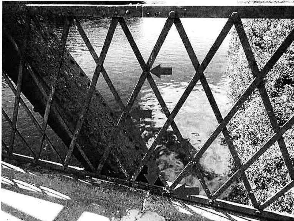
Photo 19: South sidewalk pedestrian railing at L0 - the top and bottom rail splice connections and the lattice members have missing rivets. Additionally, a lattice member to bottom rail connection bolt is loose.
