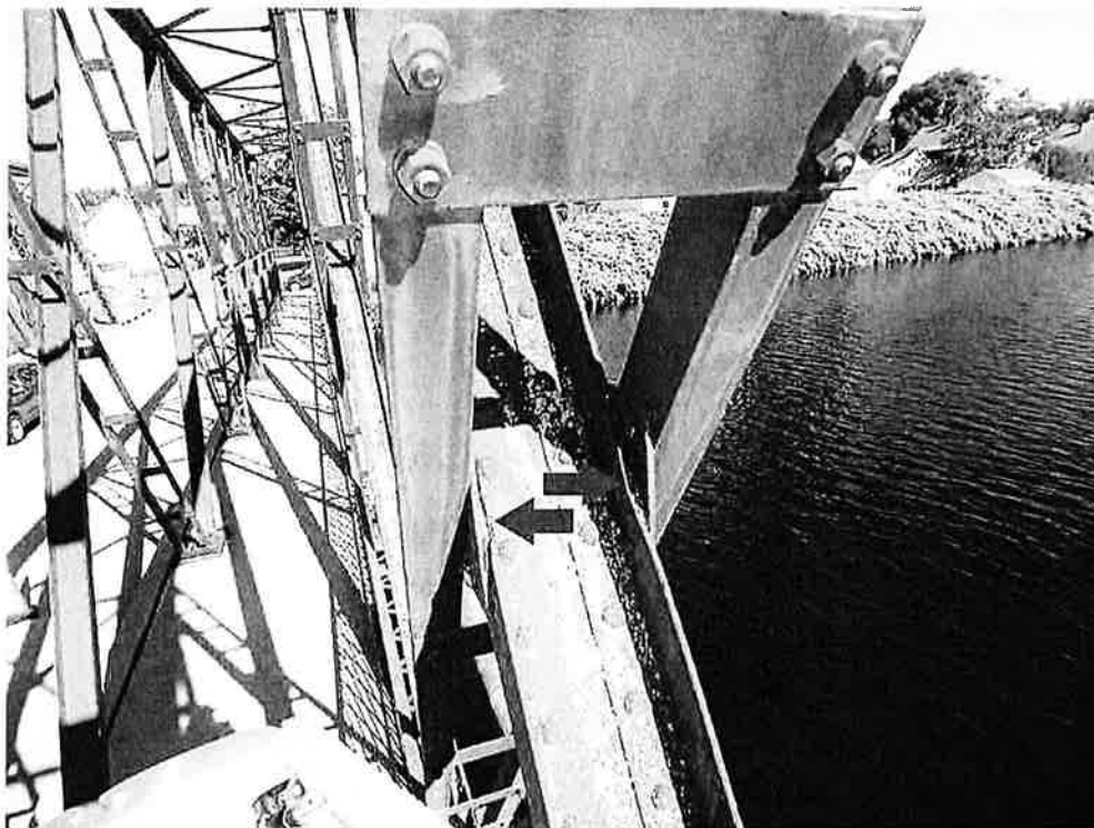
Photo 30: North tower outer truss, member U16-L14 at M15 – flanges have section loss at the edge.
