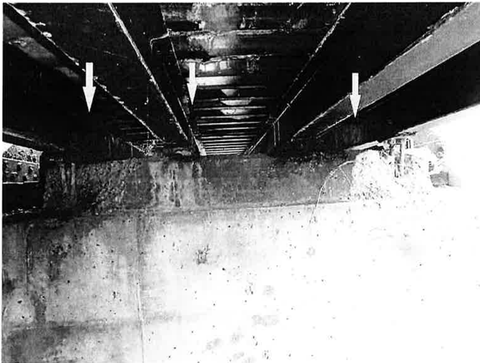
Photo 24: South sidewalk stringers at the southwest pier, looking east - peeling paint and moderate rust. Note the pedestals spalls below sidewalk stringers SW5 and SW8.
