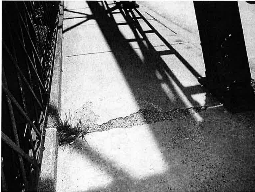
Photo 15: North sidewalk at L0, looking east - spall and vegetation growth.
