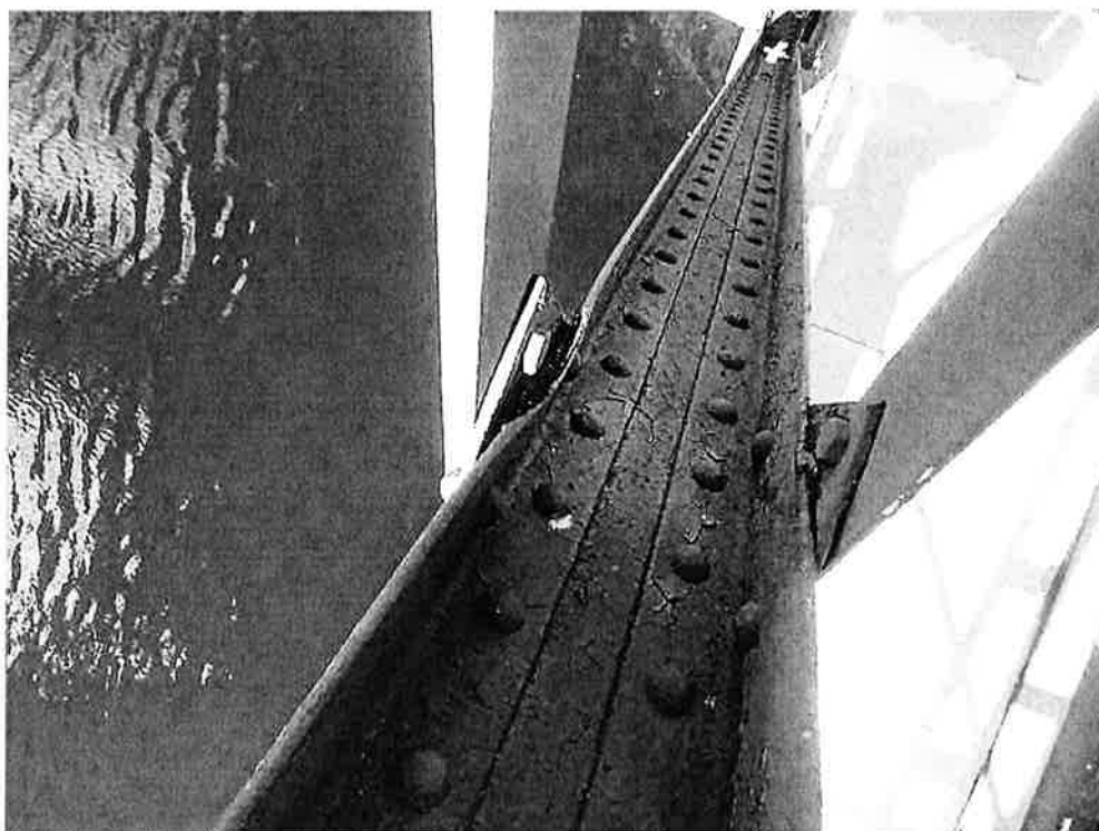
Photo 6: South tower inner truss, member U4-L2 at M3 – outer flange has section loss at the edge.
