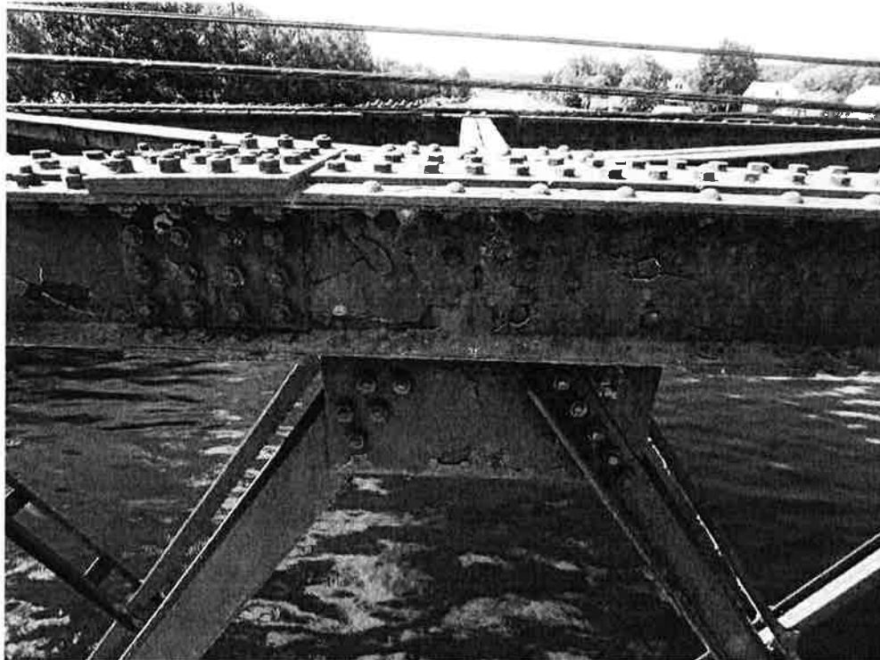
Photo 26: South tower inner truss at U12 – upper chord, lateral bracing and gusset plates with peeling paint and light rust.
