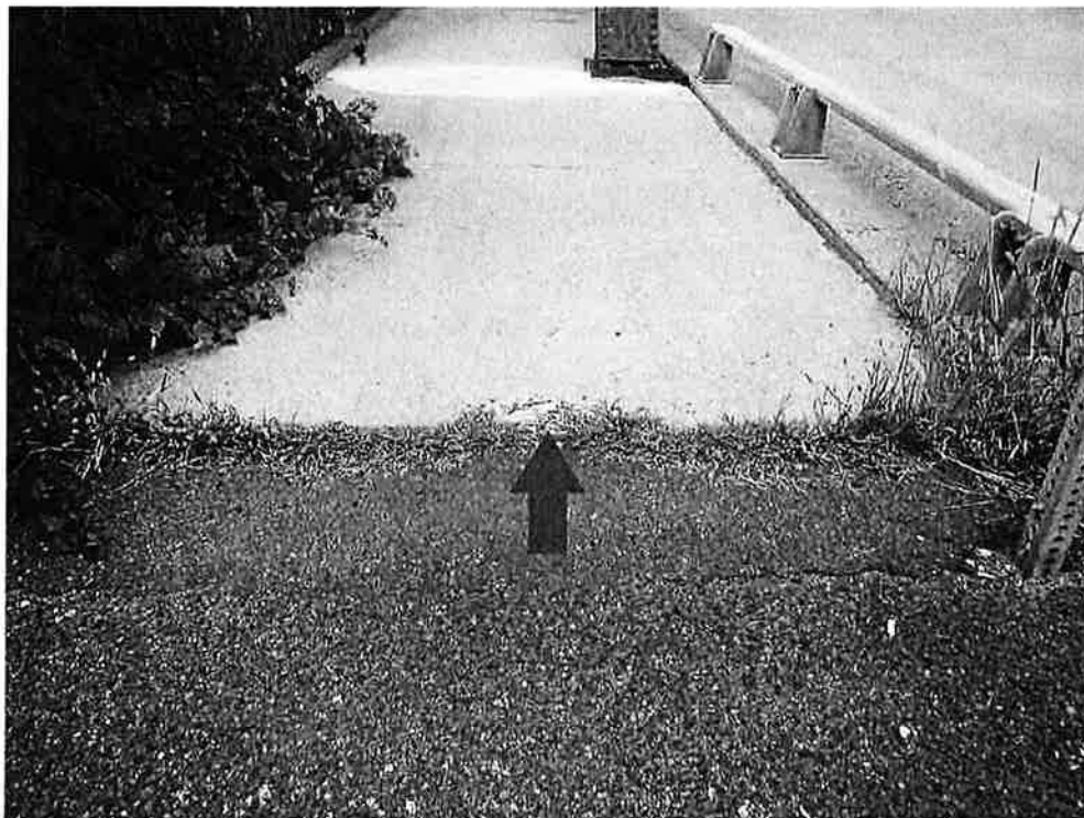
Photo 16: South sidewalk at the east end (at the interface with the southeast approach sidewalk), looking west - edge spall.
