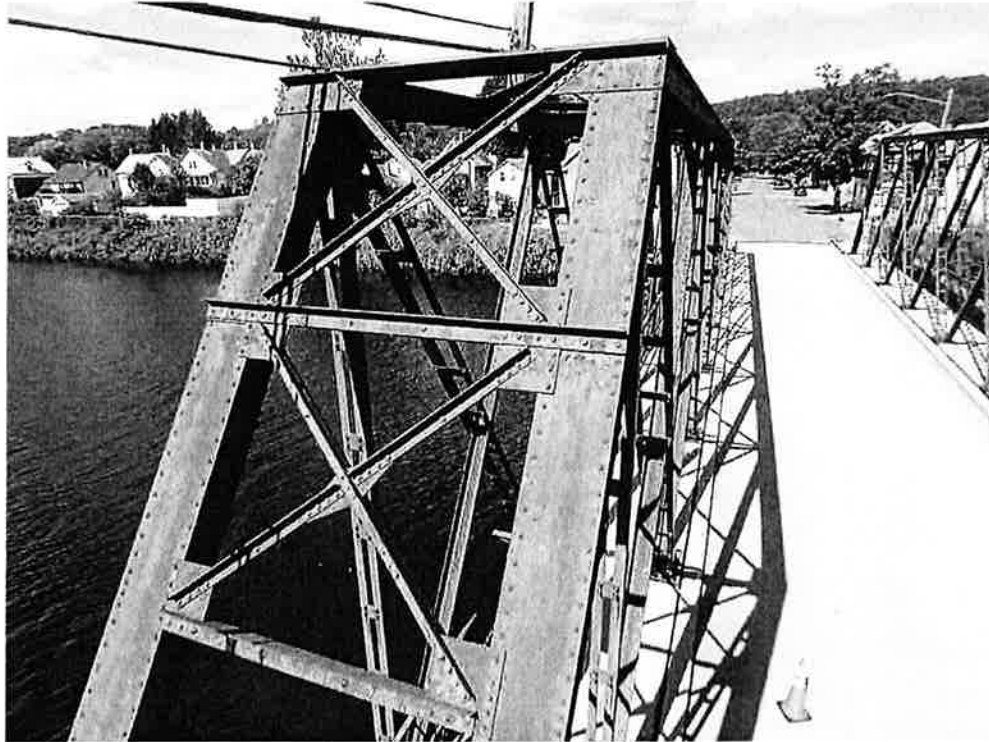
Photo 27: South truss at east portal – end posts and bracing with peeling paint and light rust.
