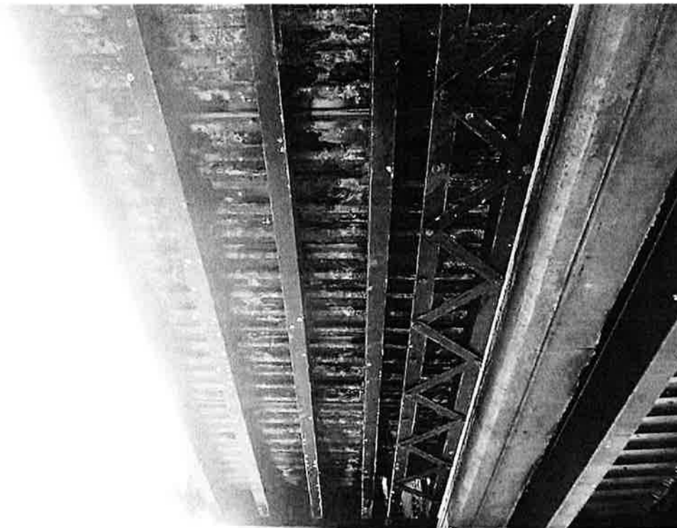
Photo 10: SIP forms, underside of south sidewalk, span 2, panel 9 (between floorbeams 9 and 10), looking west - heavy rust with isolated holes.
