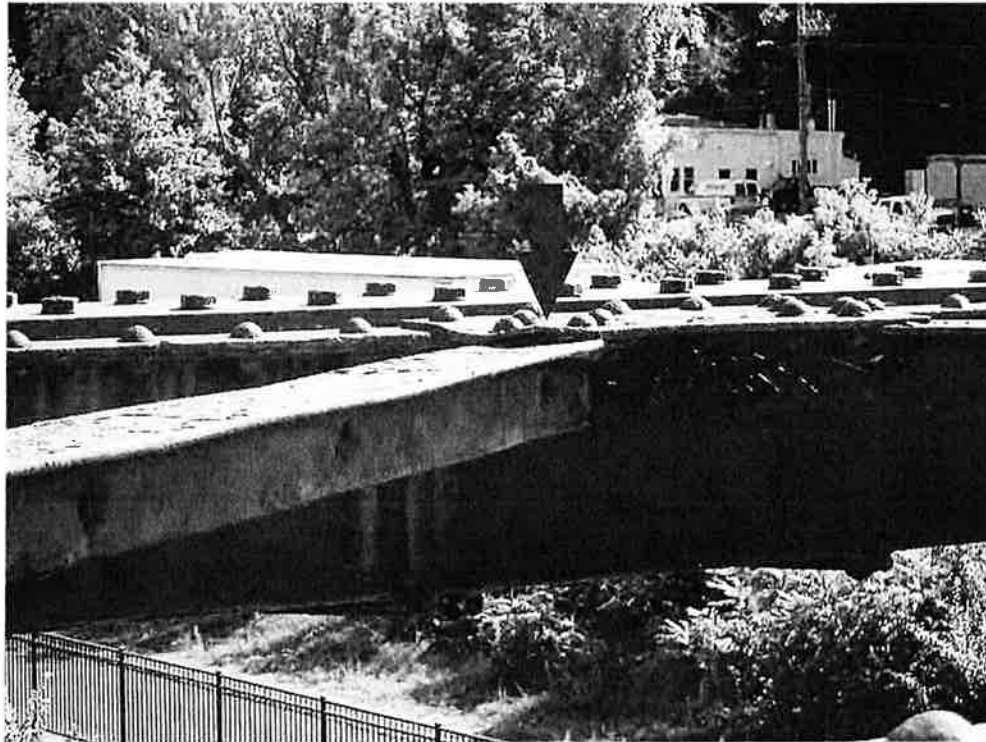
Photo 33: North tower outer truss, member U12-U14 lateral bracing connection plate - pack rust and minor bends.
