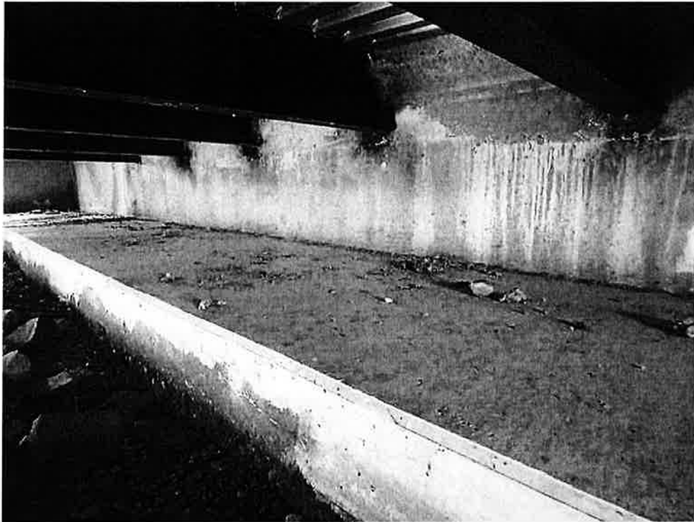
Photo 37: East abutment breastwall and backwall - scattered hairline cracks and efflorescence at the stringer ends.
