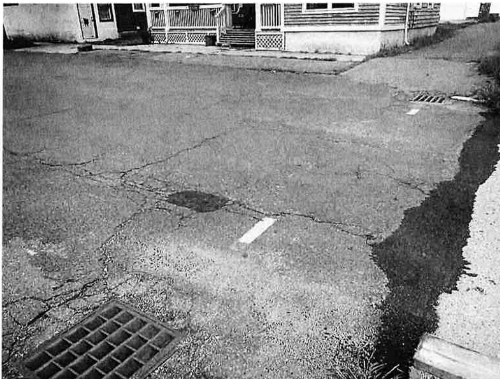
Photo 22: West approach pavement - random longitudinal and transverse cracks. Eastbound lane has a bituminous patch with adjacent area of break-up. Surrounding the drainage basins is bituminous break-up.
