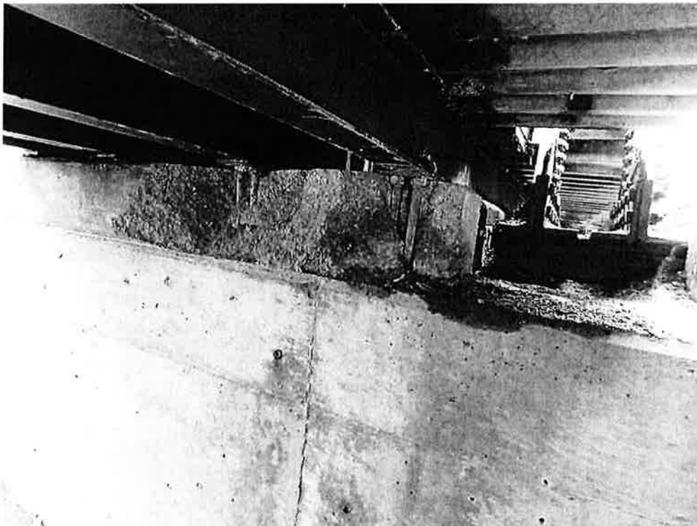
Photo 38: Northwest pier pedestal, west face, at sidewalk stringers SW3 and SW4 - spall exposing the anchor bolts and undermining the masonry plate.
