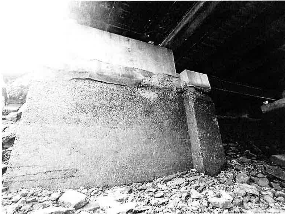
Photo 41: Northeast pier, west face – at the normal water line are spalls and hollow areas.
