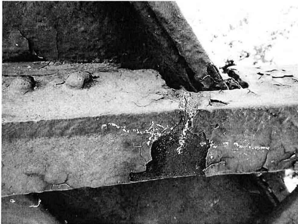
Photo 17: South sidewalk pedestrian railing, top rail, at L0-U1 - at the cut-out section is a transverse crack.
