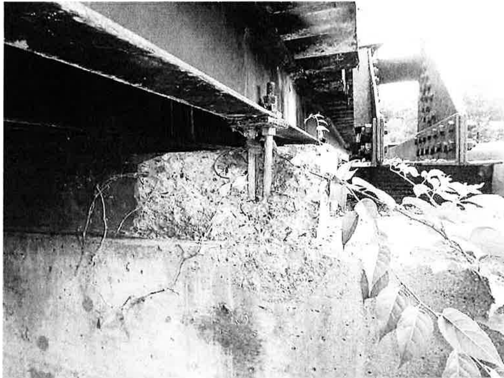
Photo 39: Southwest pier pedestal, west face, at sidewalk stringer SW8 - spall exposing the anchor rods and undermining the masonry plate.
