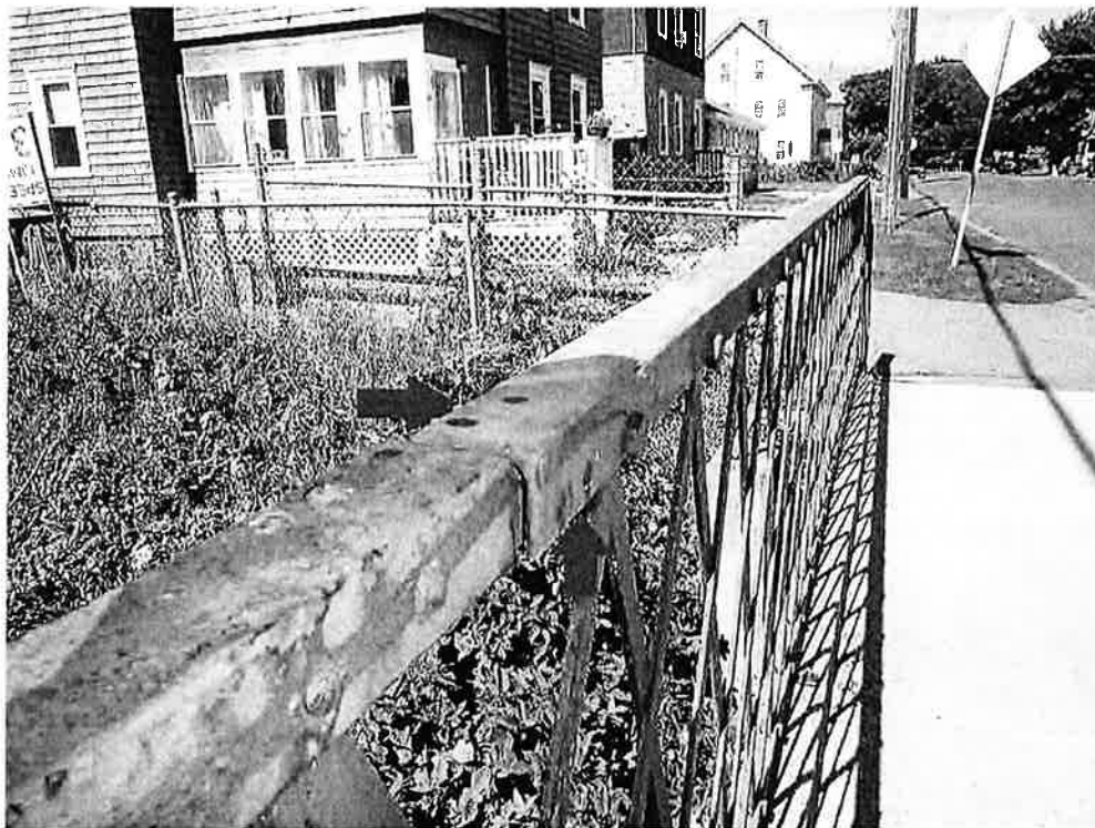
Photo 18: South pedestrian railing at L0: top rail at the splice connection is missing four (4) connection bolts and adjacent sections are laterally misaligned.
