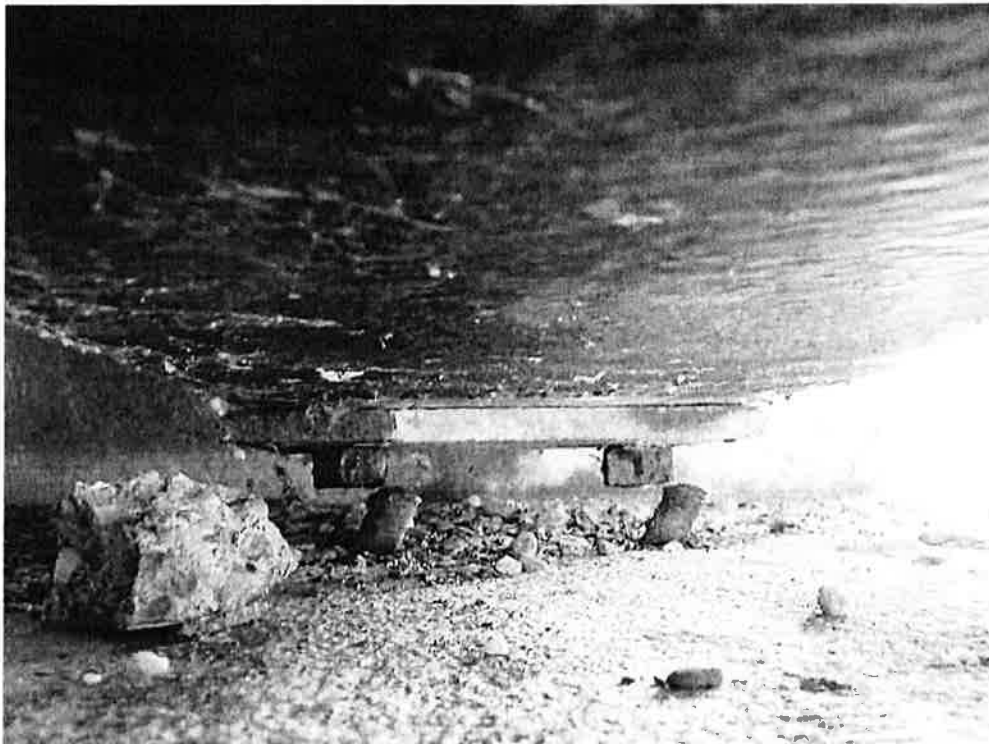
Photo 36: Northwest pier, at floorbeam 1 - both anchor rods are sheared and the floorbeam is unsupported. Note the completely spalled pedestal.
