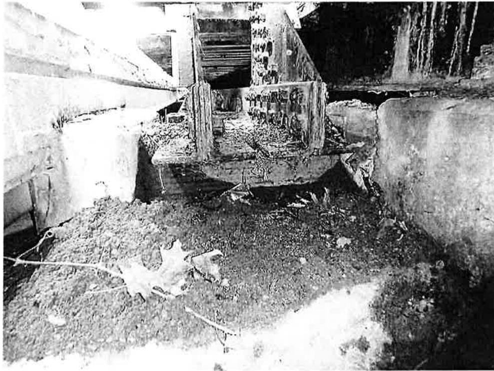
Photo 35: North tower, inner truss, east bearing - steel angles have light to moderate rust and an accumulation of debris that inhibits inspection.
