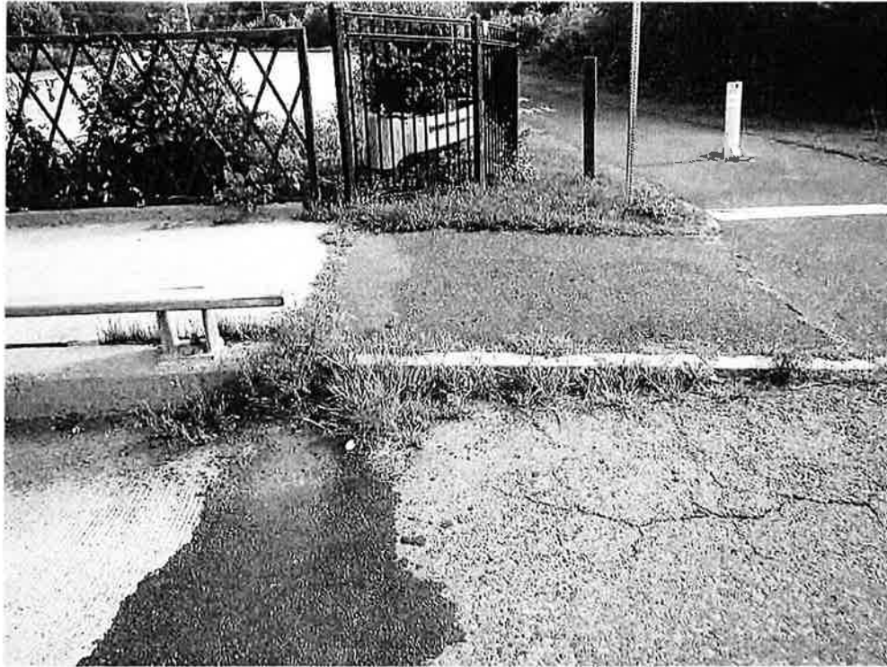
Photo 11: North curb at the east end, at the abutment saw cut - moderate vegetation growth.
