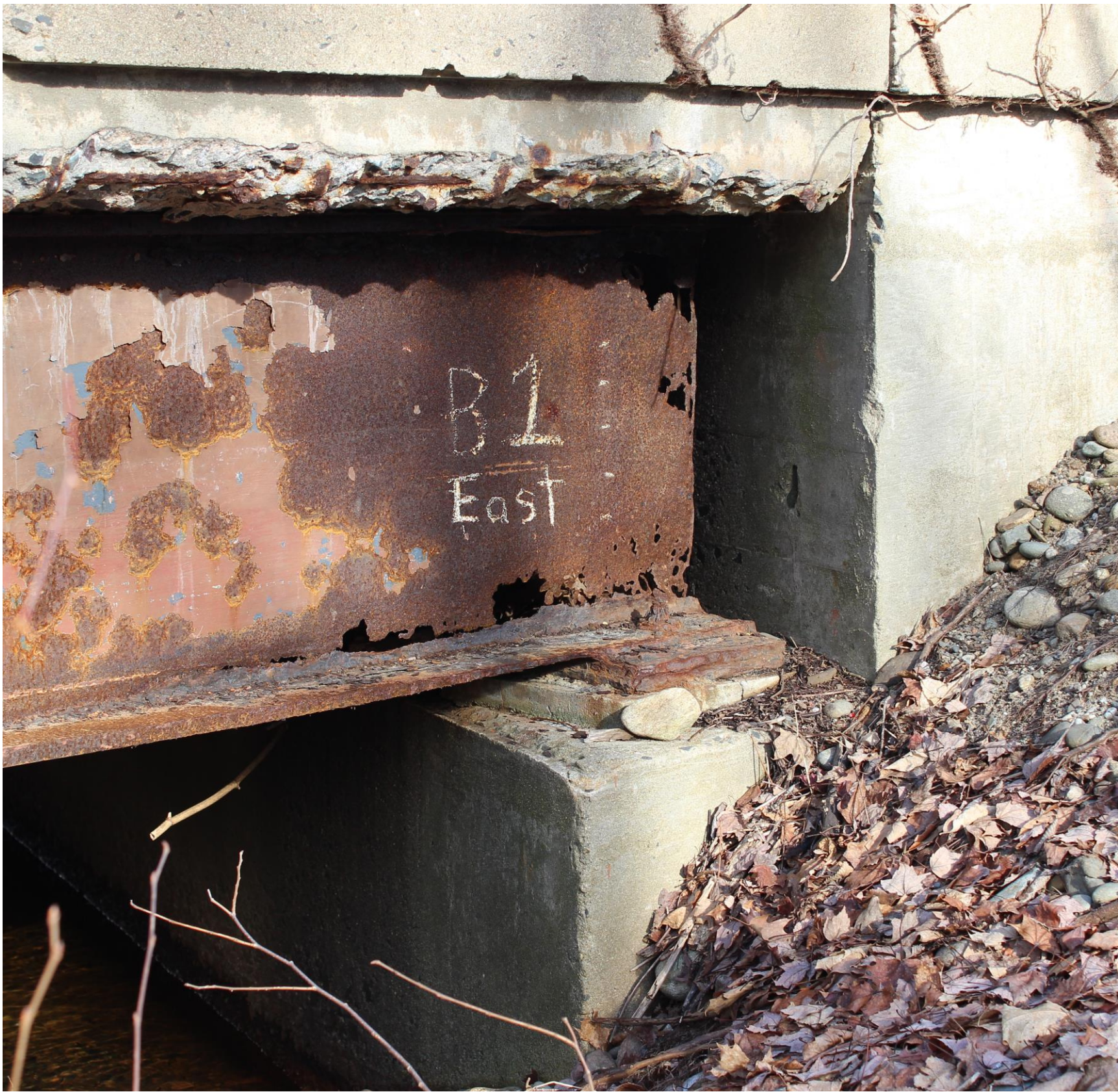
Deteriorated Superstructure
