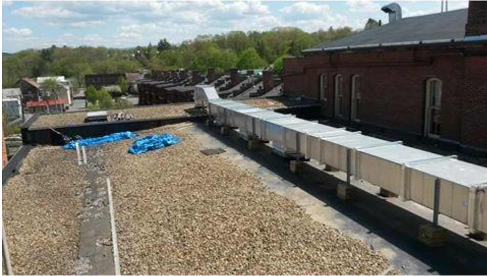
Shea Theater Upper Roof - view from Avenue A side
