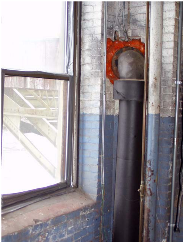
Figure 6 - 8" Water from Ped. Bridge Entering Building
