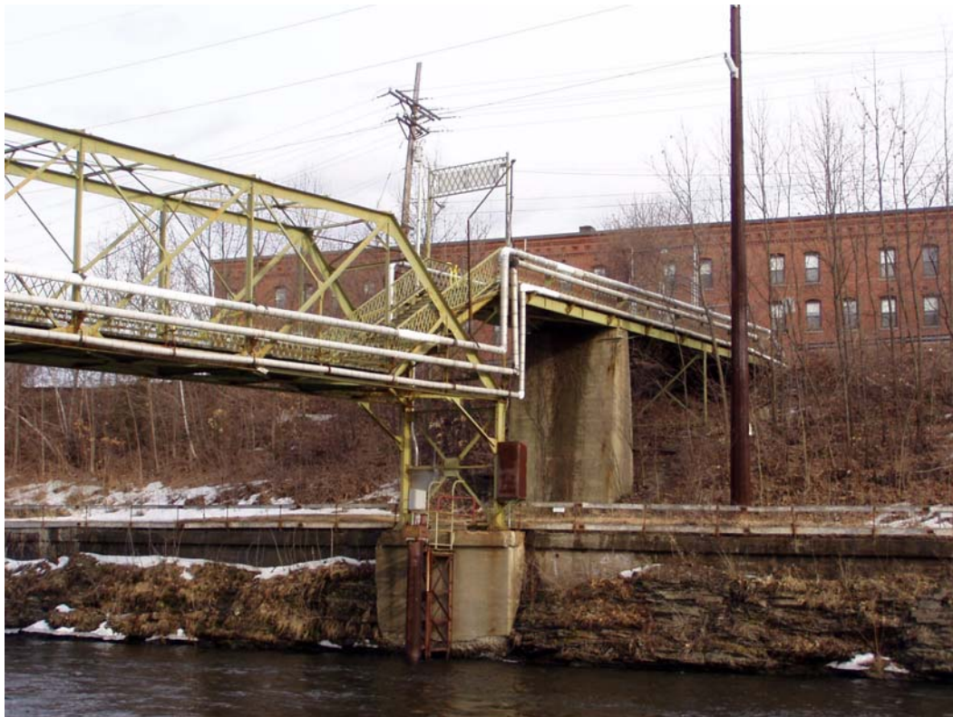
Figure 11 - Utilities Crossing Pedestrian Bridge
