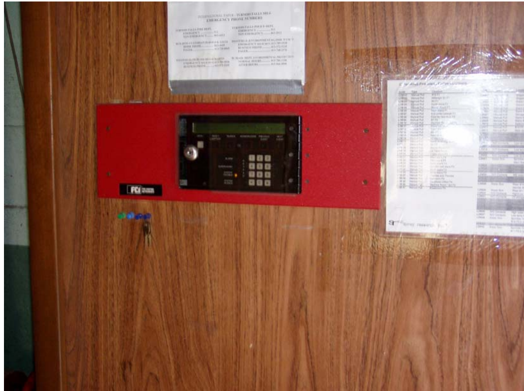
Figure 8 - Fire Alarm Panel
