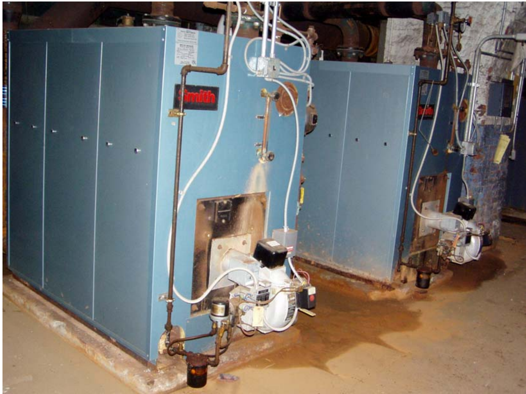
Figure 5 - Newer HB Smith Boilers
