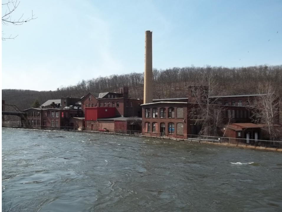
Photograph 1. Strathmore Mill looking northwest.
