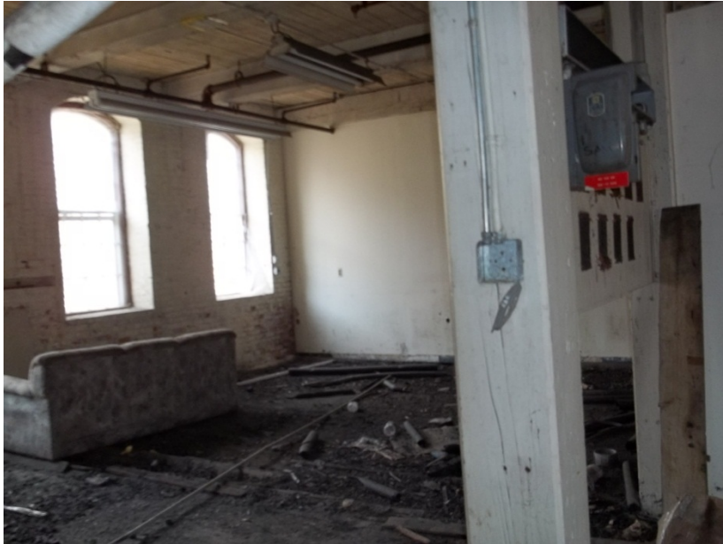
Photograph 3. Interior of mill building.
