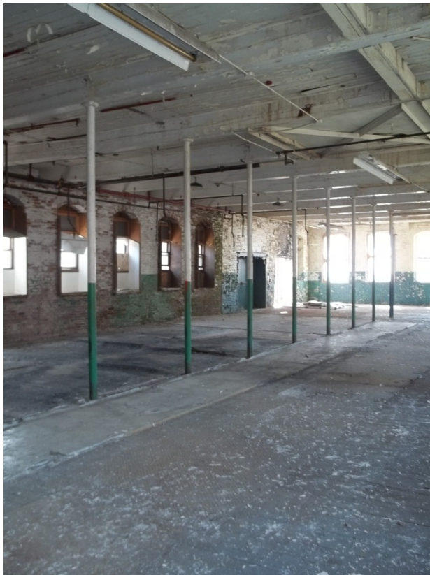
Photograph 2. Interior of mill building.
