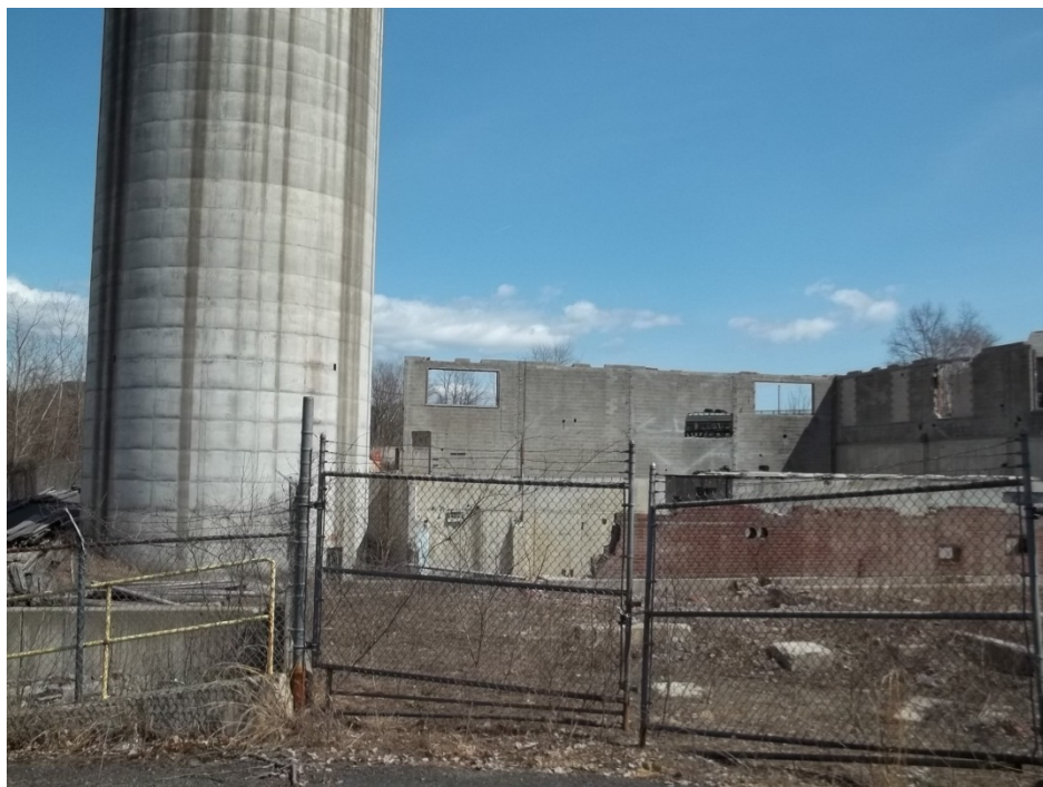
Photograph 5. Former Indeck facility on east side of site.
