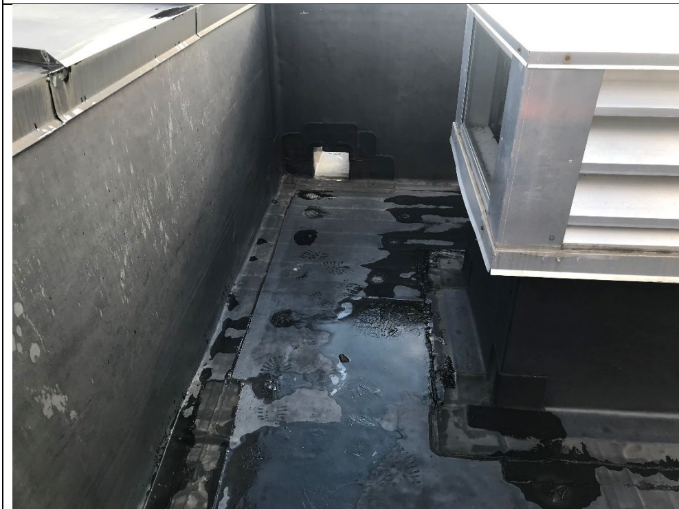
Photo R12 01/06/22 Photo Location: Rear Stairwell Roof Description: View of vent over elevator chase and second through wall scupper at base of parapet.
