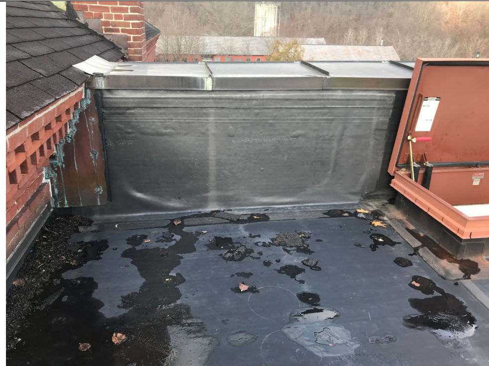
Photo R9 01/06/22 Photo Location: Rear Stairwell Roof
