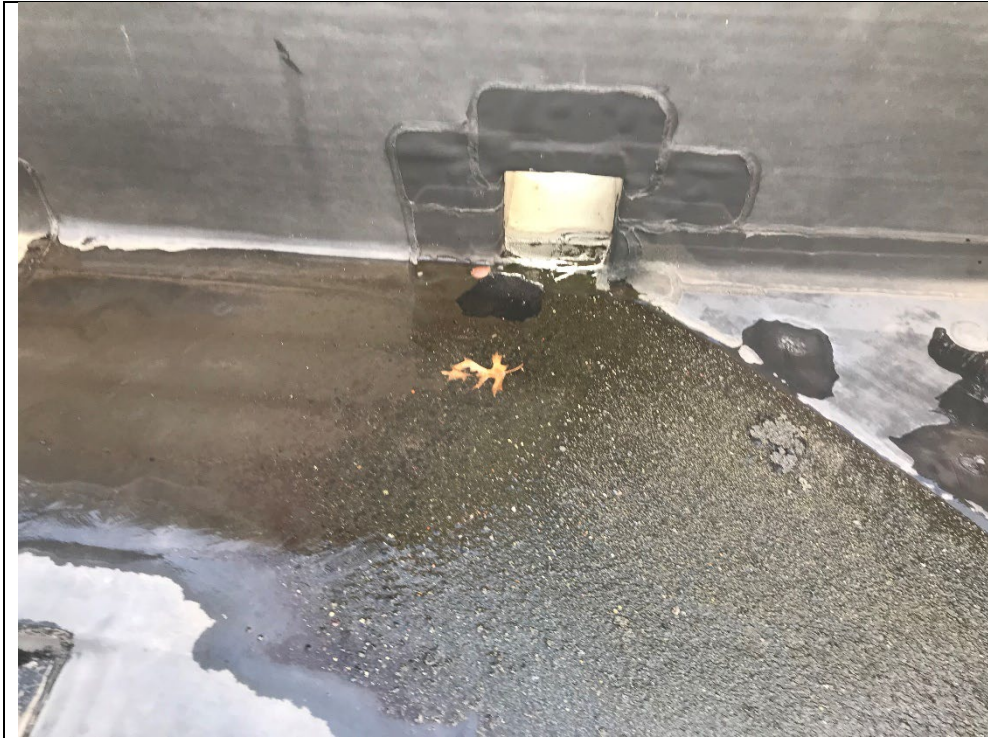
Photo R11 01/06/22 Photo Location: Rear Stairwell Roof Description: Debris accumulating around through wall scupper in parapet.
