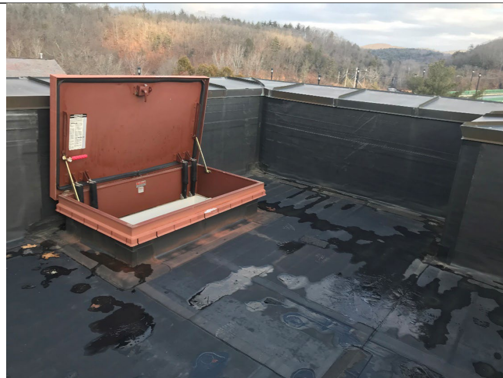
Photo R10 01/06/22 Photo Location: Rear Stairwell Roof
