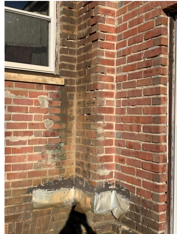
Deterioration of northwest inside corner of the 1900 Building
